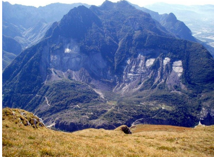
Figure 7.15: View of the mount Toc in the present days, with vegetation on the surface of the slide.
