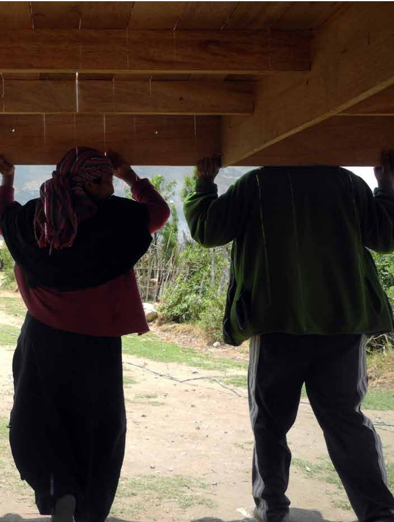
Photo: Floating modules' structure transportation, construction site, Cachiviru.
