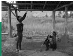
13 th of JUNE 2015 Survey on site
