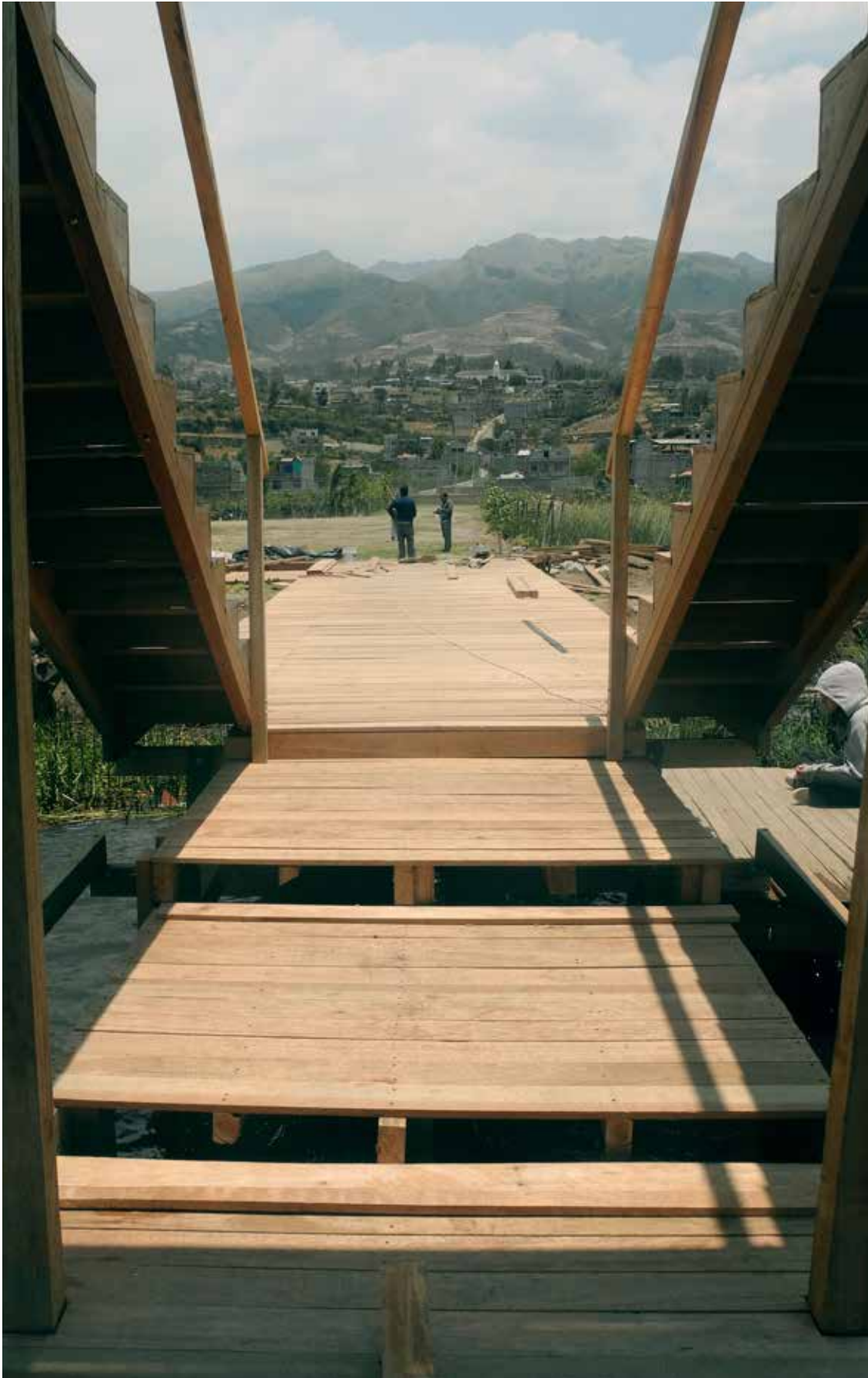
Photo: Boardwalk and stairs- view from below, construction site, Cachiviru.
