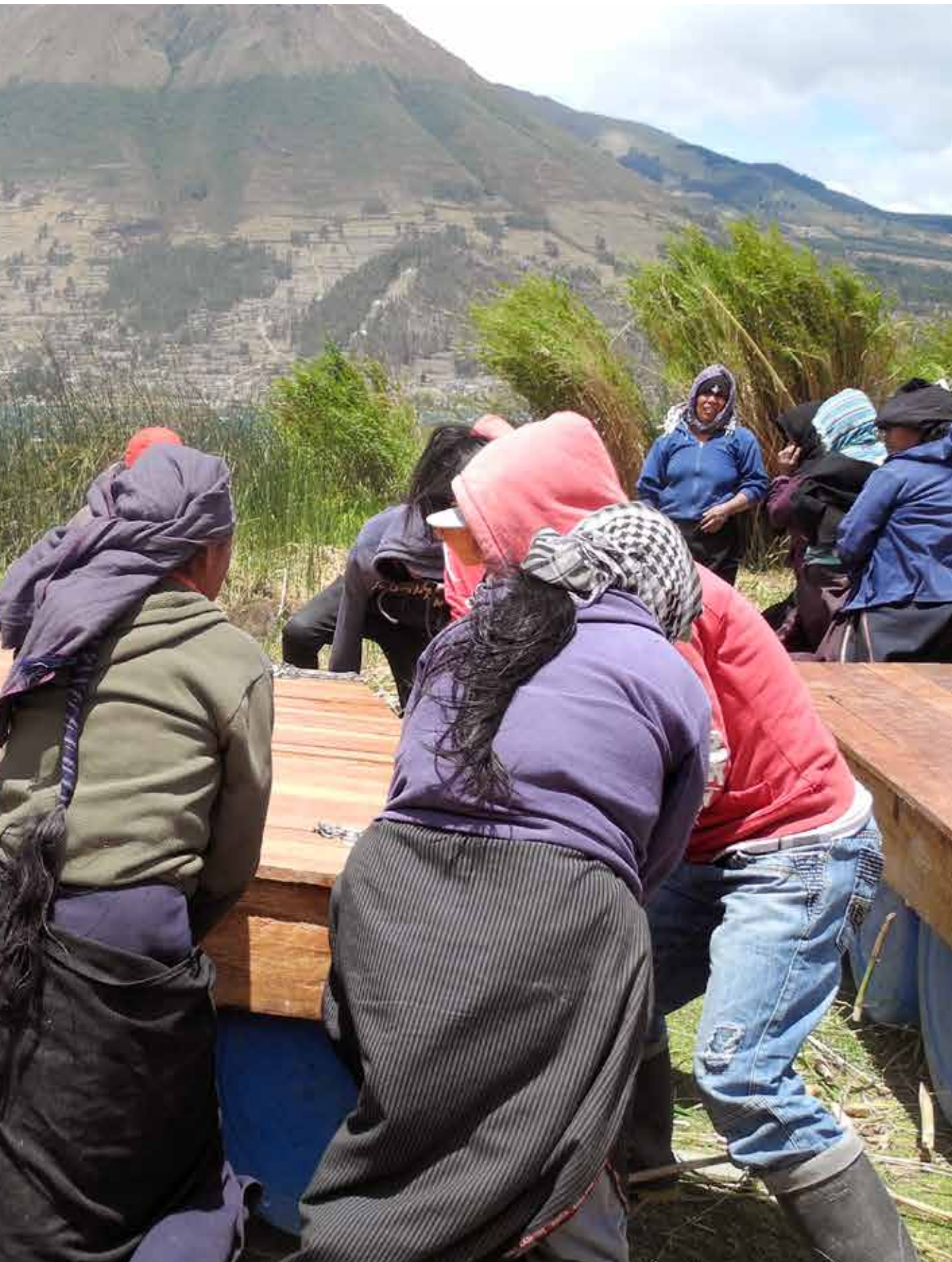
Photo: Community transporting floating modules into the water, construction site, Cachiviru.
