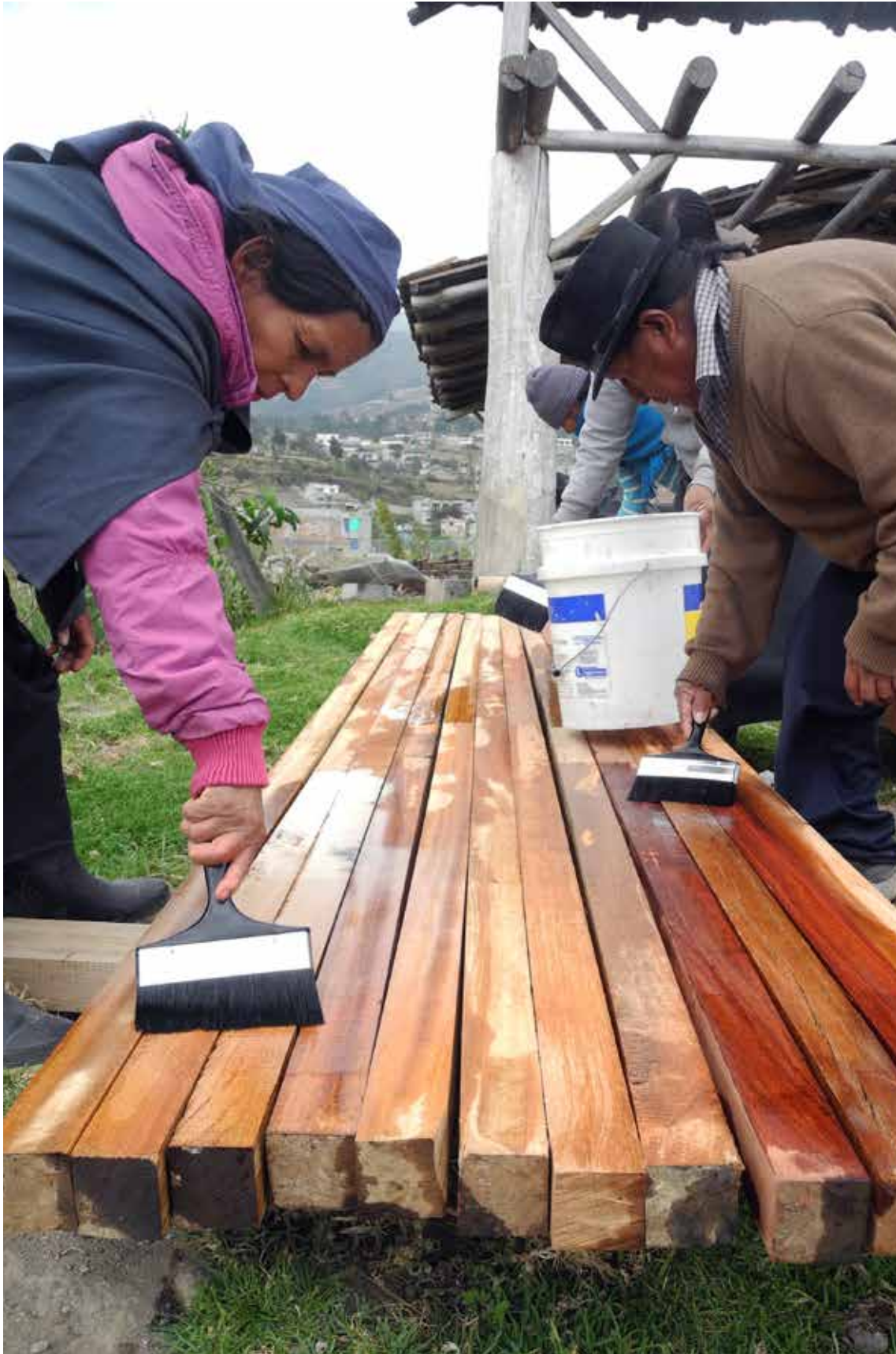
Photo: Belen and Marlon varnishing wood, construction site, Cachiviru.
