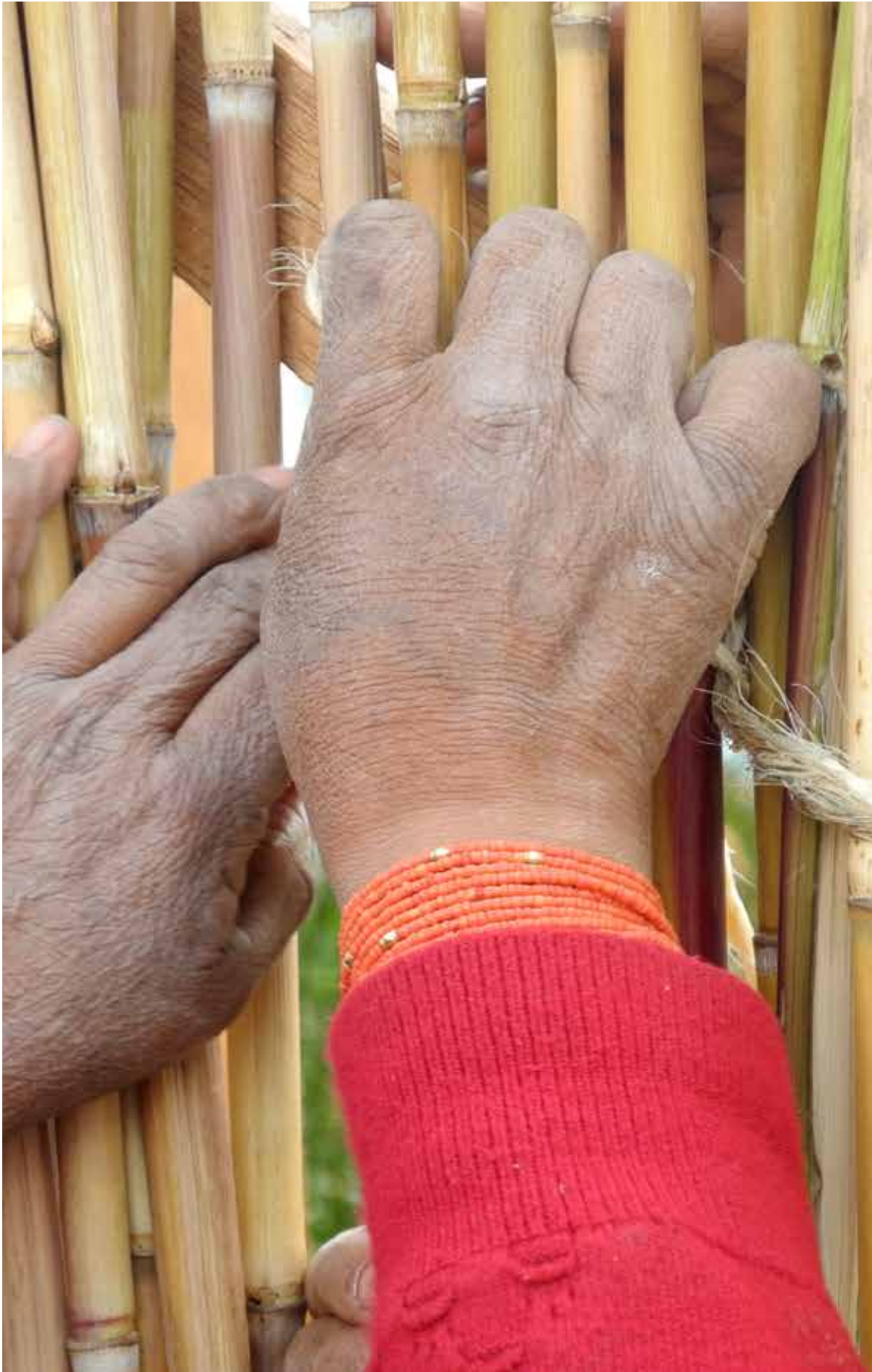
Photo: hands tying carrizo, construction site, Cachiviru.
