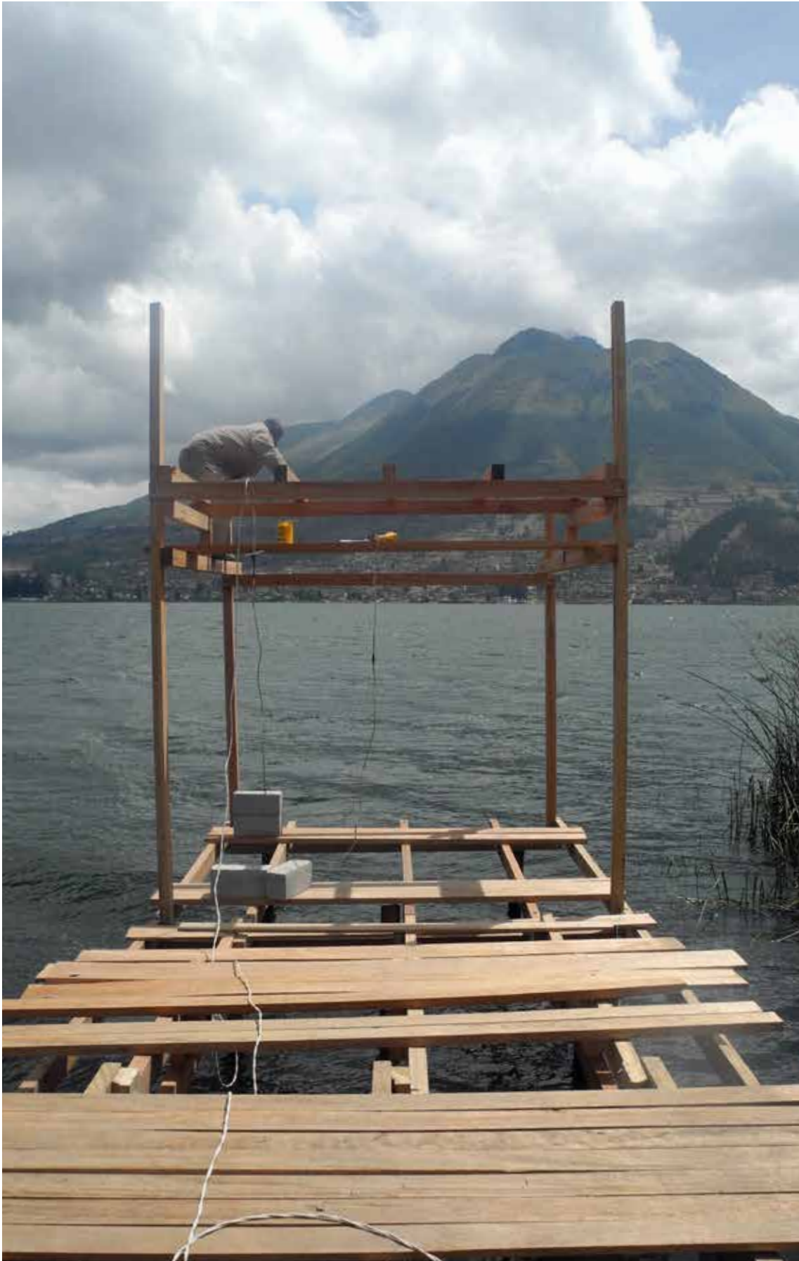
Photo: Wilson working on Mirador structure, (safe) construction site, Cachiviru.
