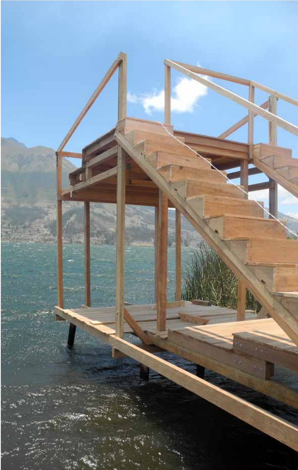
Photo: Mirador structure - lateral view, construction site, Cachiviru.
