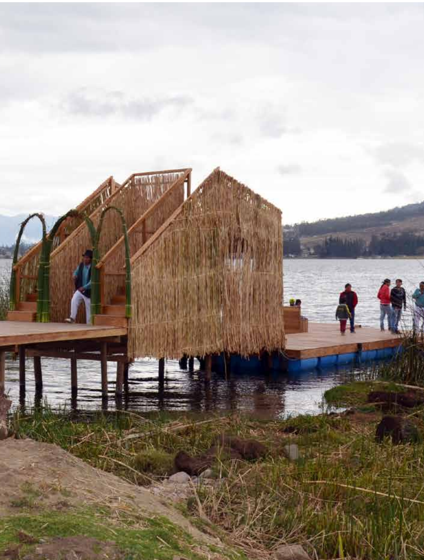
Photo: Muelle-Mirador - lateral view from the Lake's shore, Cachiviru.
