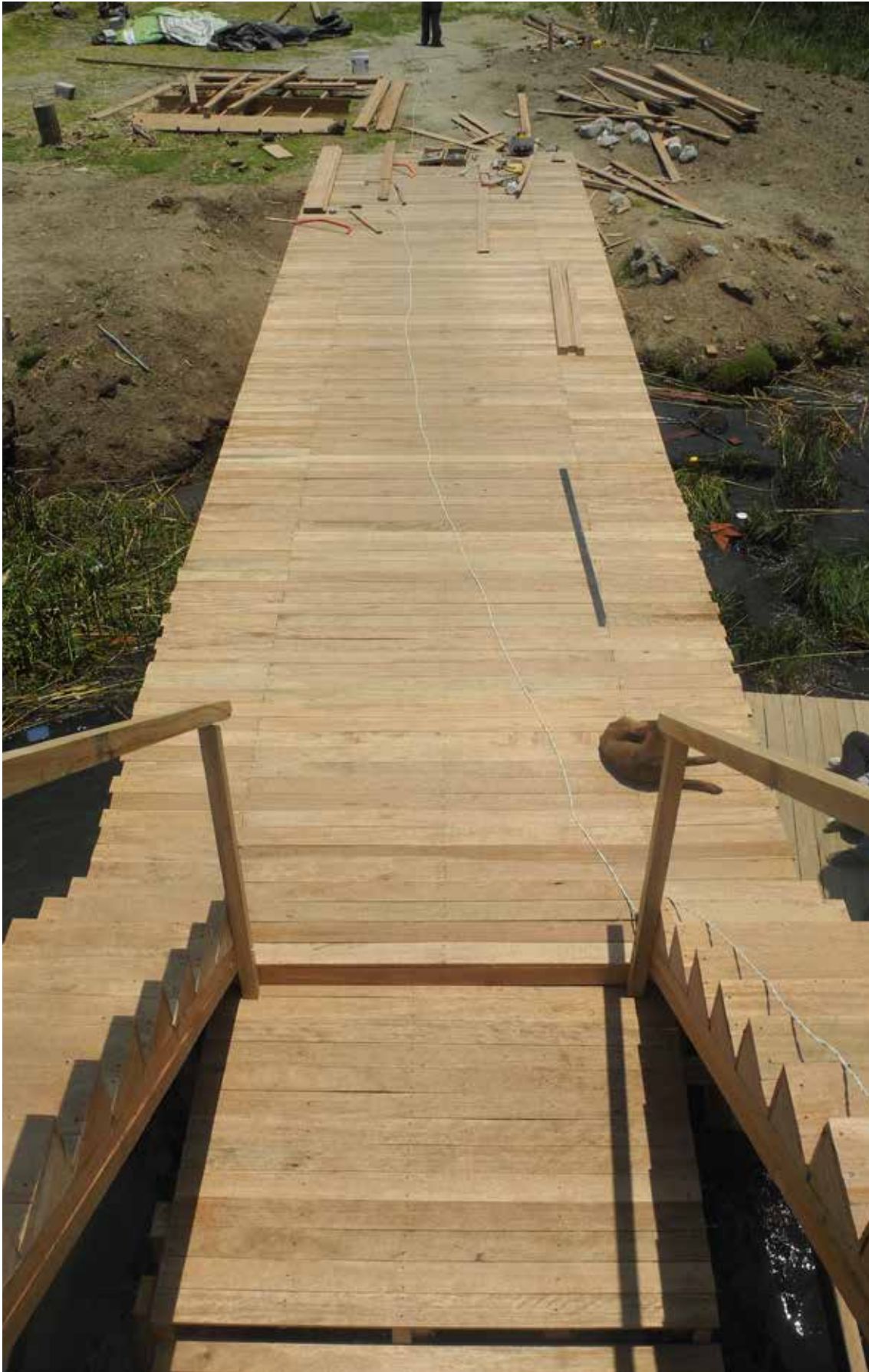
Photo: Boardwalk - view from the Mirador, construction site, Cachiviru.
