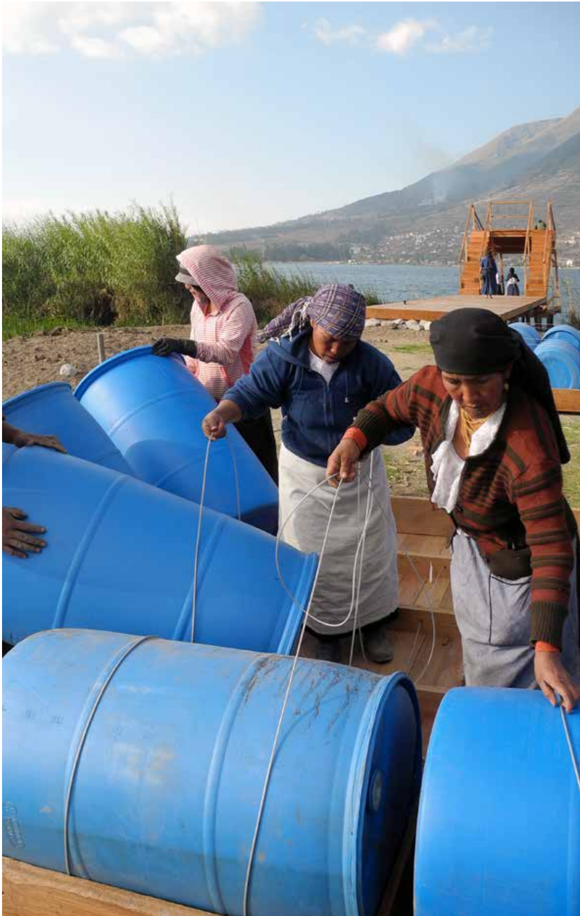
Photo: Maria, Pilar and Carmen tying tanks, construction site, Cachiviru.
