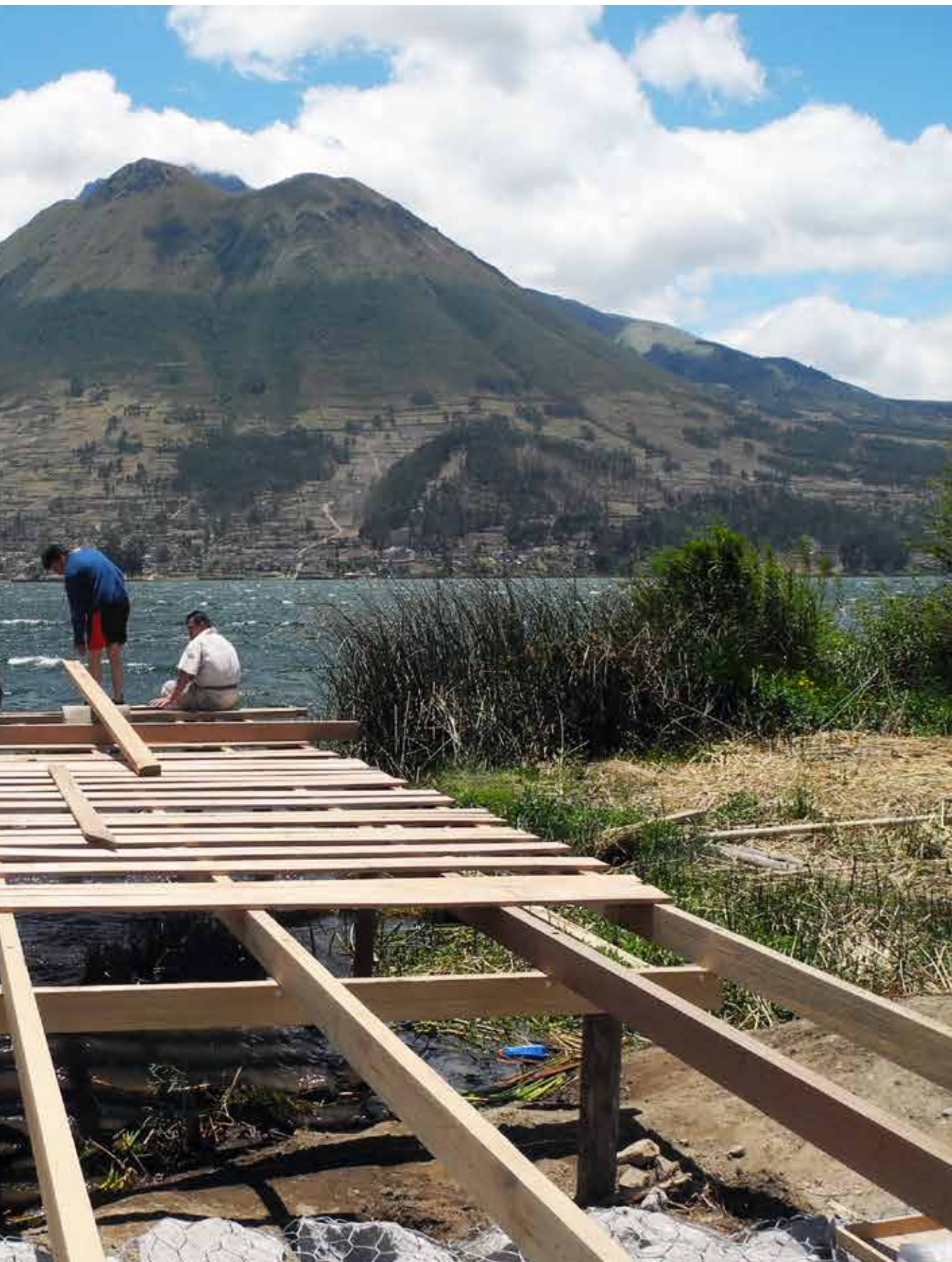
Photo: Construction site situation - week 2: carpenters working on boardwalk structure, Cachiviru.
