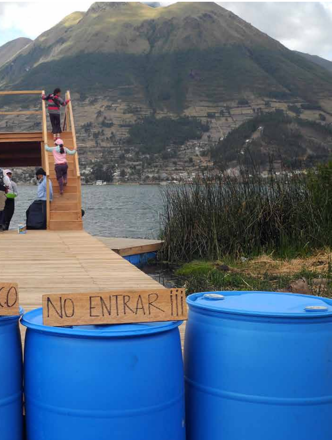
Photo: Construction site situation - week 5: "wet varnish, do not enter!" , Cachiviru.
