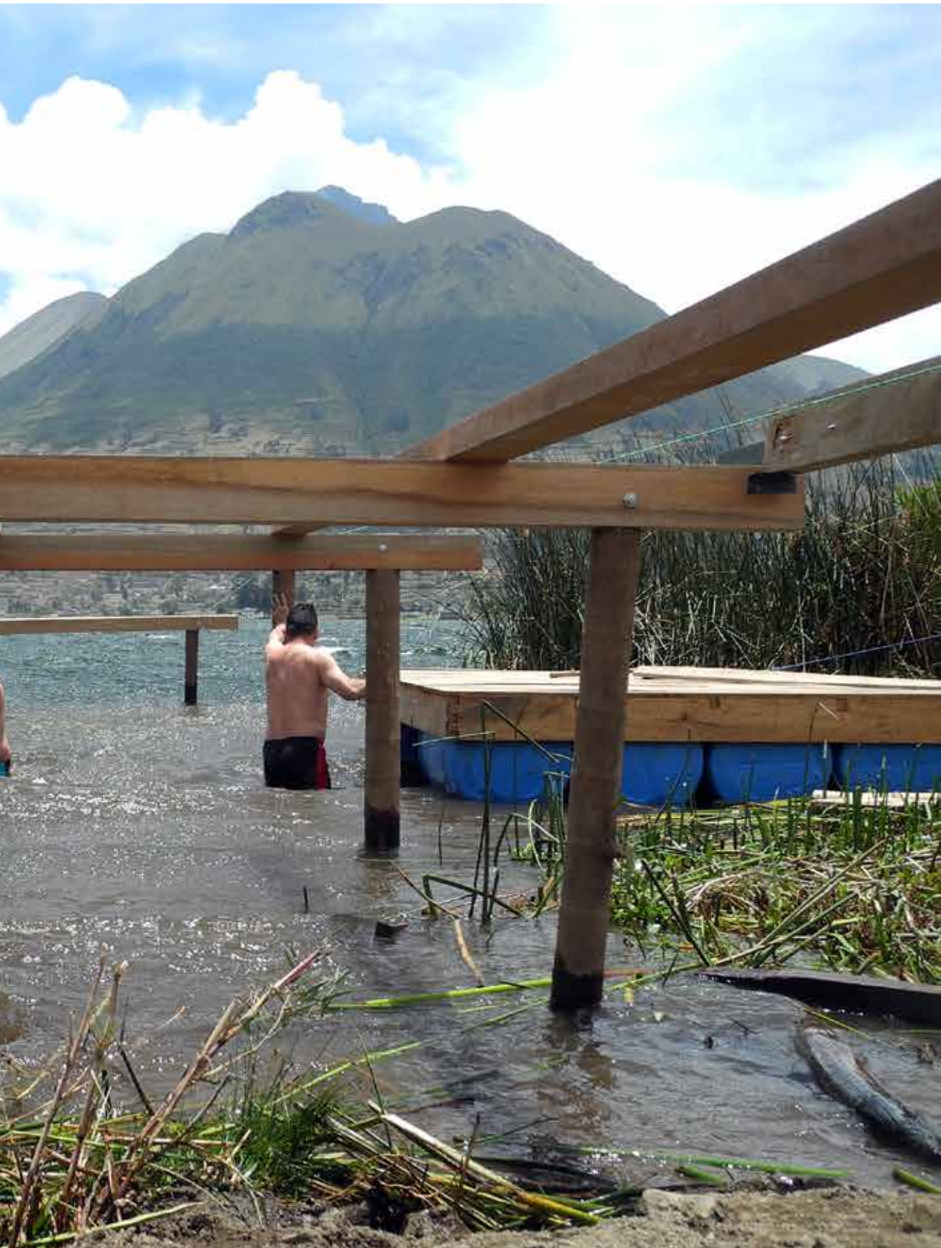
Photo: Santiago and Wilson working on foundations-beams' stabilization, construction site, Cachiviru.
