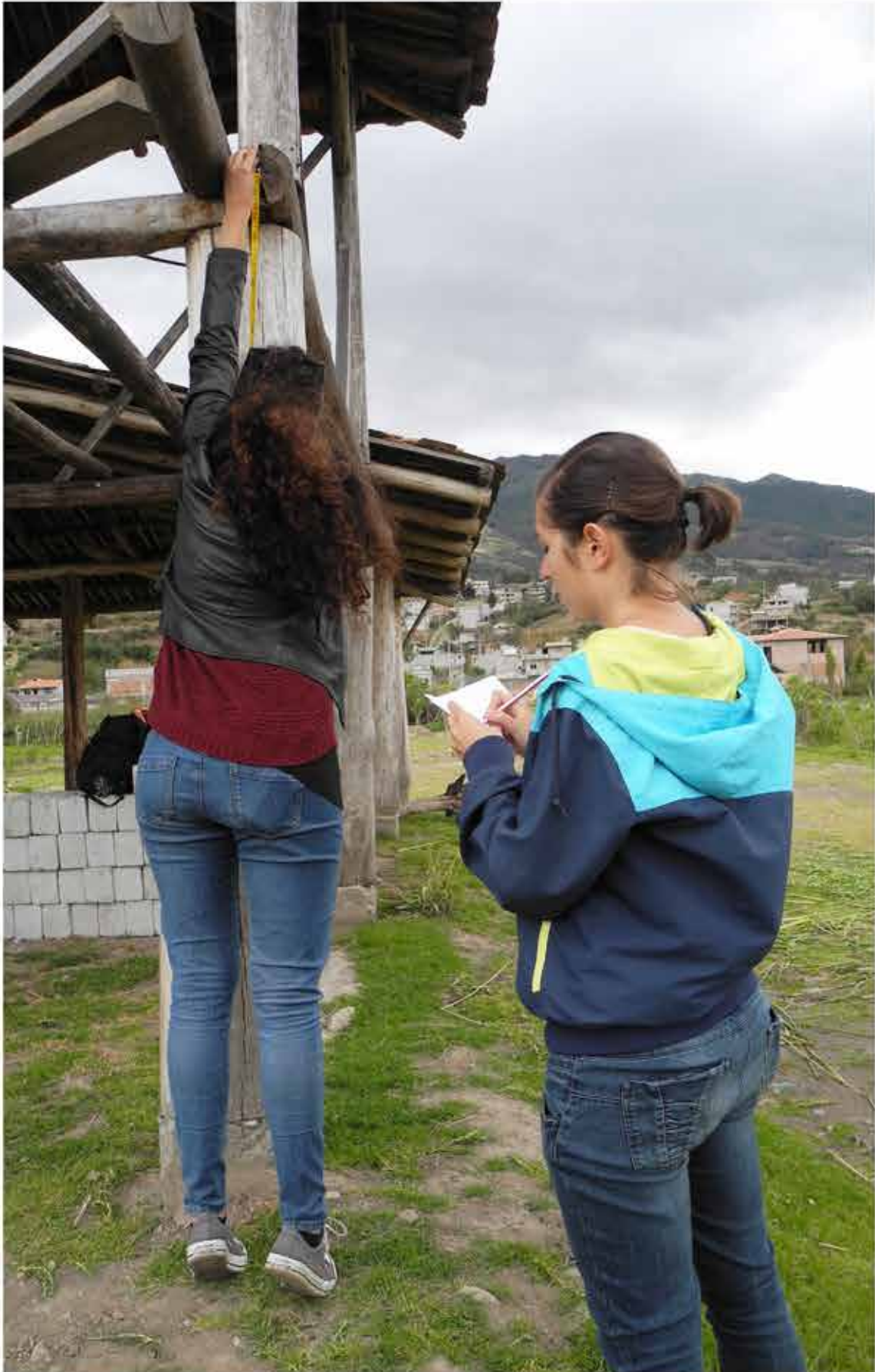
Photo: Measurement of the existing wooden structure beams and their diameters
