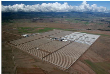
Figure 1.2: The Andasol solar power station is 150-megawatt (MW) concentrated solar power station and Europe first commercial plant to use parabolic troughs.
