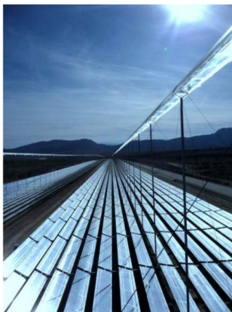
Figure 1.4: The PE1 has been the first Fresnel-lens, solar power plant connected to the grid, in March 2009
