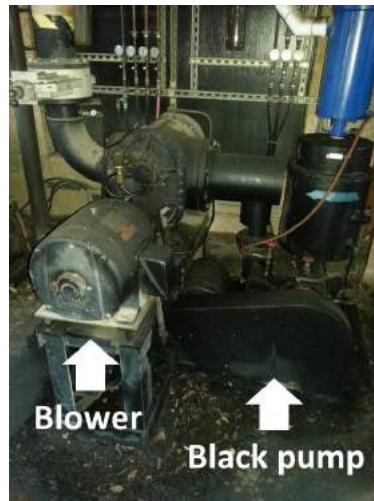
Figure 3.2: Roughing pumps
