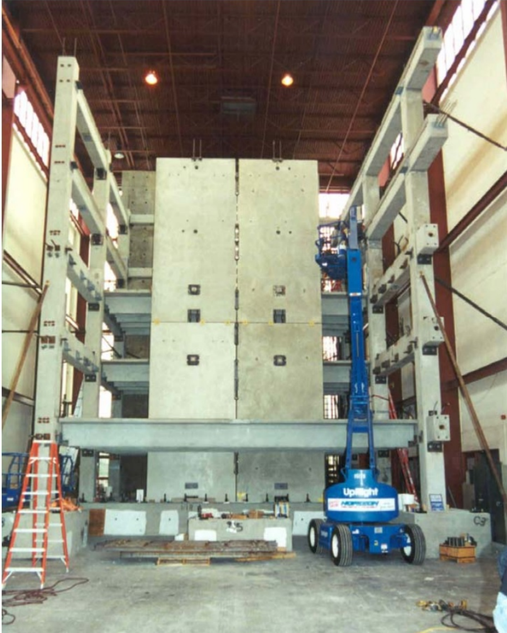
Figure 4.6: Erection of the unbonded post-tensioned jointed precast wall
