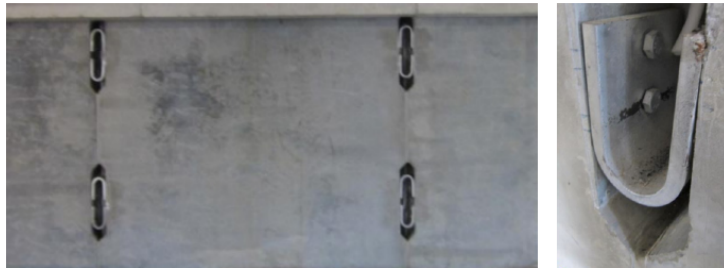
Figure 3.9: U-shaped flexural plate (UFPs)
