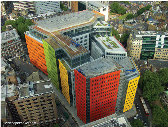
[200] Central Saint Giles, 2007-2010 R. Piano, London Hosting offices and residences in the center of the city, the Architect wanted to build a social more than functional center, giving lots of space to the always busy public areas, and that could become a nevralgic point for the neighbourhood with its ground and roof gardens.
