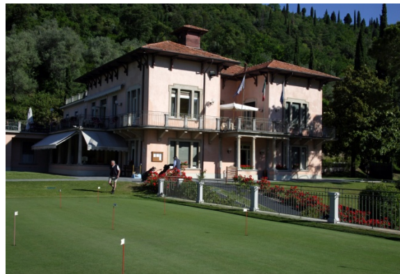
Figura 79: 2008 club house e putting green
