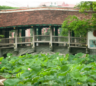
Figura 4.18 Pond Bridge, Hanoi
