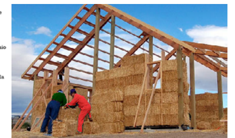
Figura 3.21 Infill bale walls
