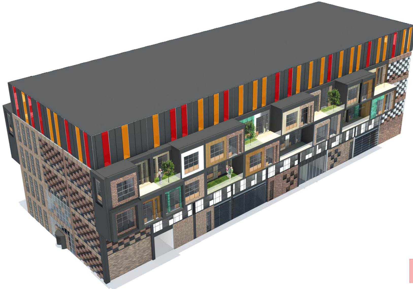
Standard 5-storey block with possibility to hang 1/3 part of prefabricated module on the facade as cantilever
