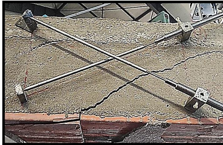
Figure 33. Failure of the second consolidated floor slab of h = 12 + 5 cm. (Source: Laboratory image)
