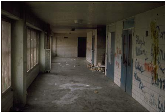
Figure3-2 Interior of Pruitt-Igoe
