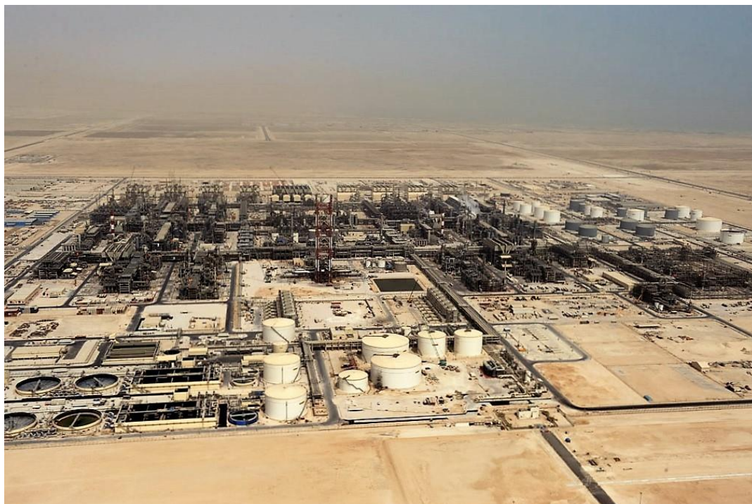
Figure 1.33: Aerial view of Pearl GTL plant [42]
