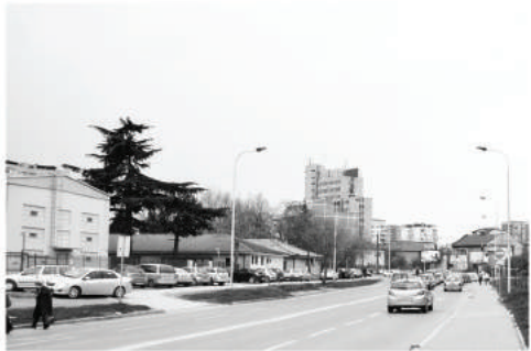
Barracks of factory for Tabacco
