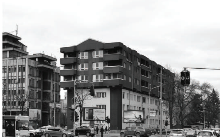
3. Added floors to preexisting building
