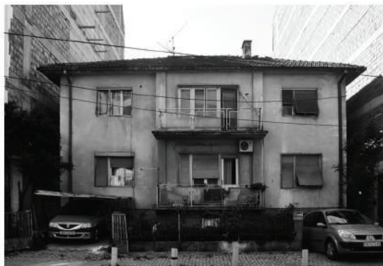
26. Remained house in-between two residential buildings
