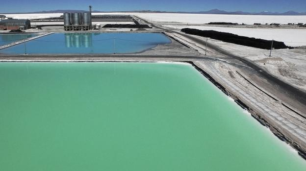
Lithium brine deposits are accumulations of saline groundwater that are enriched in dissolved lithium. This process is as follows, brine, typically carrying 200–1,400 milligrams per liter (mg/l) Li, is pumped to the surface and concentrated by evaporation in a succession of artificial ponds, each one in the chain having a greater Li concentration.
