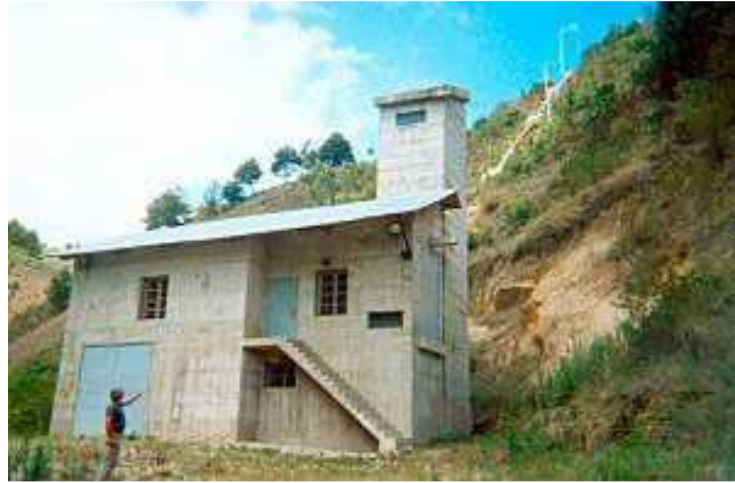
Figure 2-3 Reservoir micro hydro plant of Bomalang'ombe
