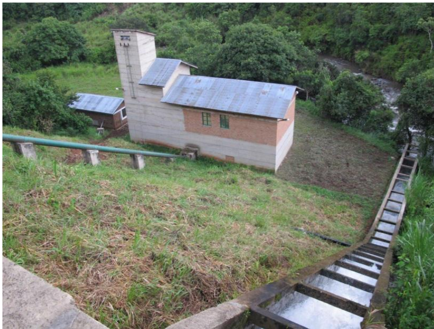
Figure 2-4 Run-of-the-river micro hydro plant of Ikondo
