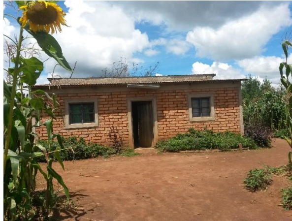
Figure 4-6 Typical house in rural villages
