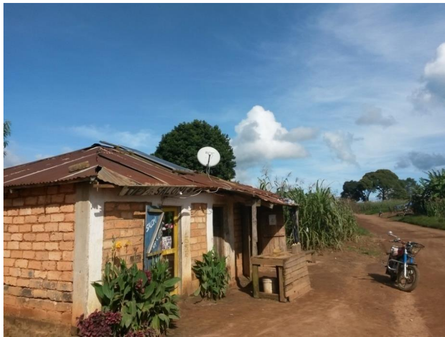
Figure 3-5 Hair Cutter connected to Solar Home-based system
