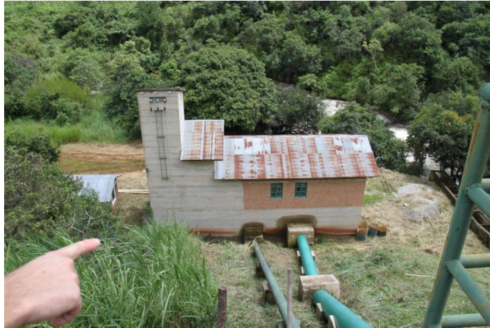
Figure 2-5 Run-of-the-river micro hydro plant upgraded in Ikondo
