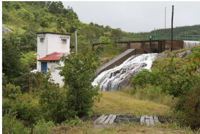
Figure 2-2 Reservoir micro hydropower plant of Matembwe
