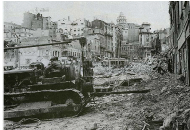
Menderes demolitions Salt research archive.
