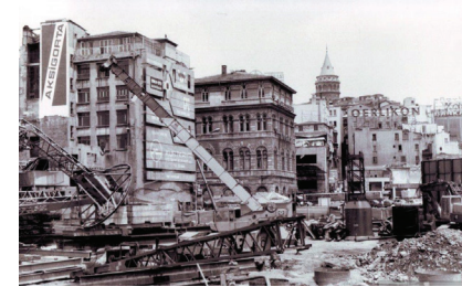
Dalan demolitions. Salt research archive.
