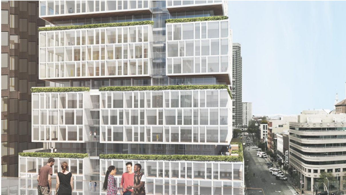
Figure 60: View onto the face, where the column distribution is not visible from the outside (Source: Courtesy of SOM, 2015)
