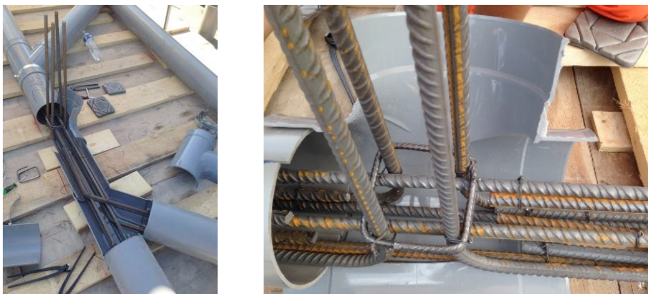
Figure 2.21: Density of reinforcement.
