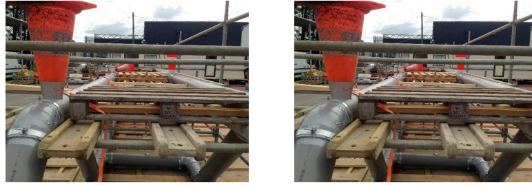
(a) Concreting step.
