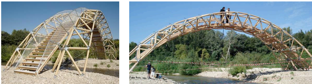
Figure 2.2: Paper Bridge structure.
