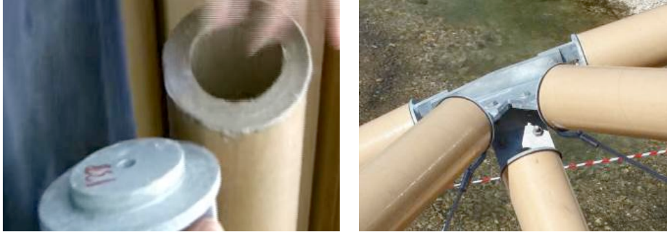
Figure 2.3: Paper Bridge. Details of the connections.
