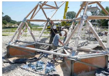
(b) Provisional shoring.
