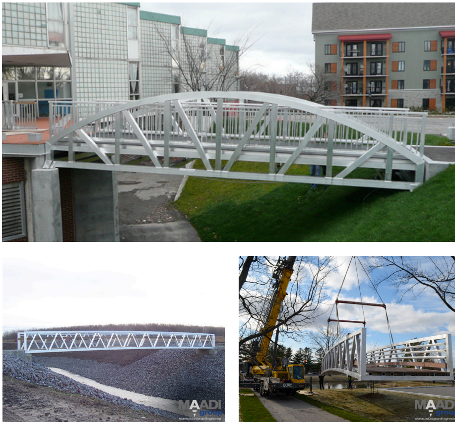
(b) Prefabricated bridges by Maadi.
