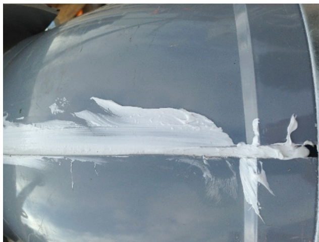
Figure 2.22: Liquid seal to avoid concrete leaks.
