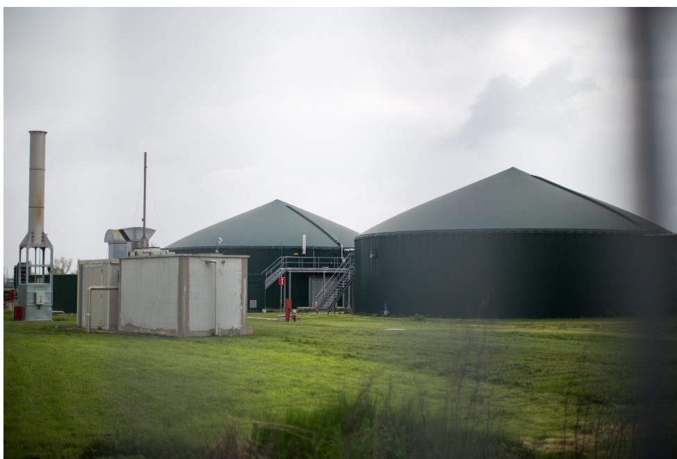
Figure 5-2: A view of two main digester, flare and CHP unit into "Azienda Agricola Codeluppi", situated in Campegine (RE).
