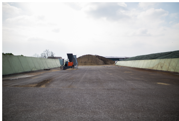
Figure 5-24: Solid Fraction of post digestate storage area in “Azienda Agricola San Prospero”.
