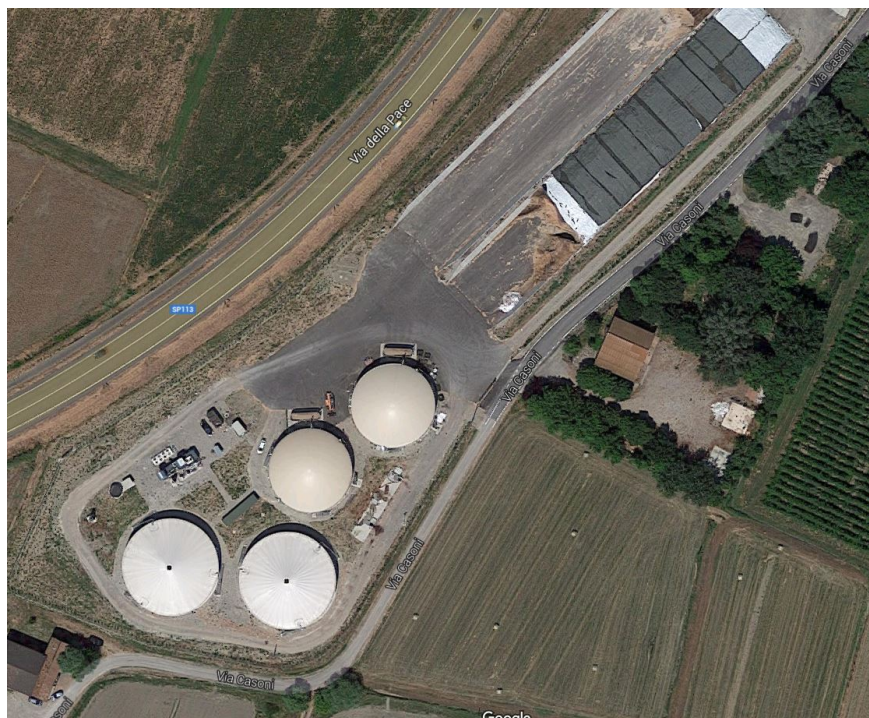
Figure 5-13: A Satellite view of the biogas plant on Gazzata (RE). It is immediate to understand layout simplicity with only two digesters and respective digester tanks. No separator and no post digester are present. (Source: Google Earth)
