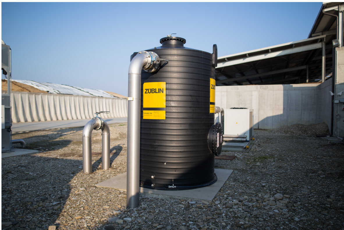
Figure 5-11 : Activated Carbon Filter used as pre-treatment process in order to decrease H 2 S biogas content
