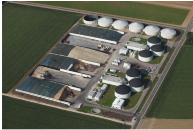
Figure 4-19: Plienigen Biogas Plant
