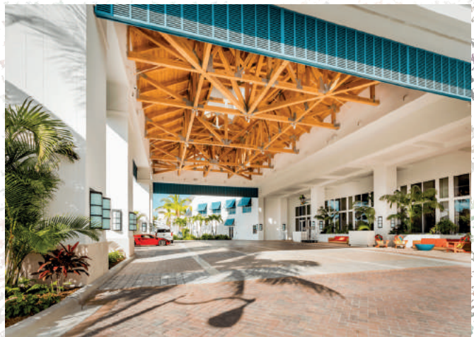
Figure 2.2.8 Entrance, Margarita ville Hollywood Beach Resort, Florida, USA, 2016
