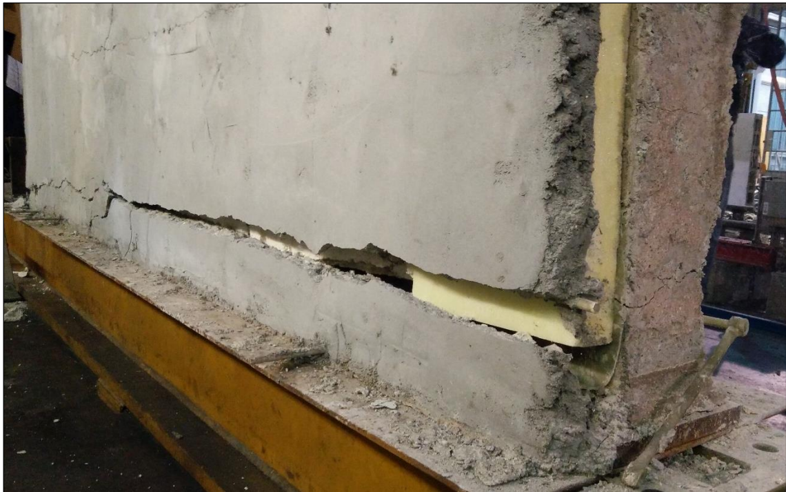
Figure 5-9. Sixth loading cycle – uplift of the infill
