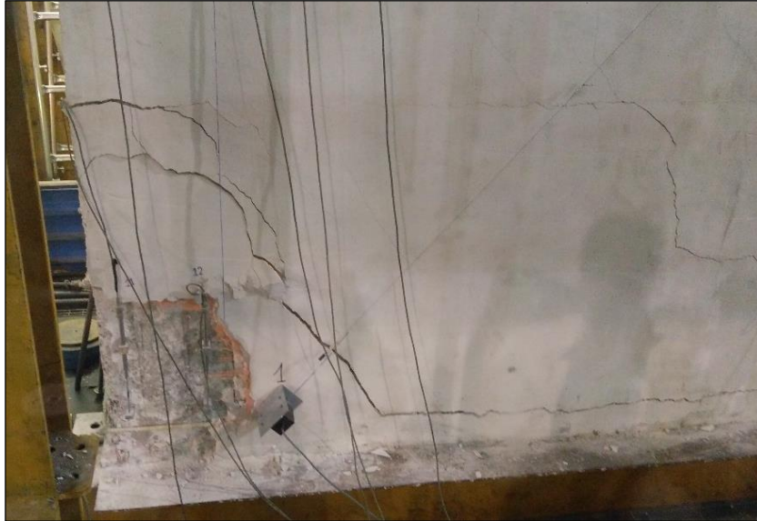
Figure 5-3. New cracks during the third cycle
