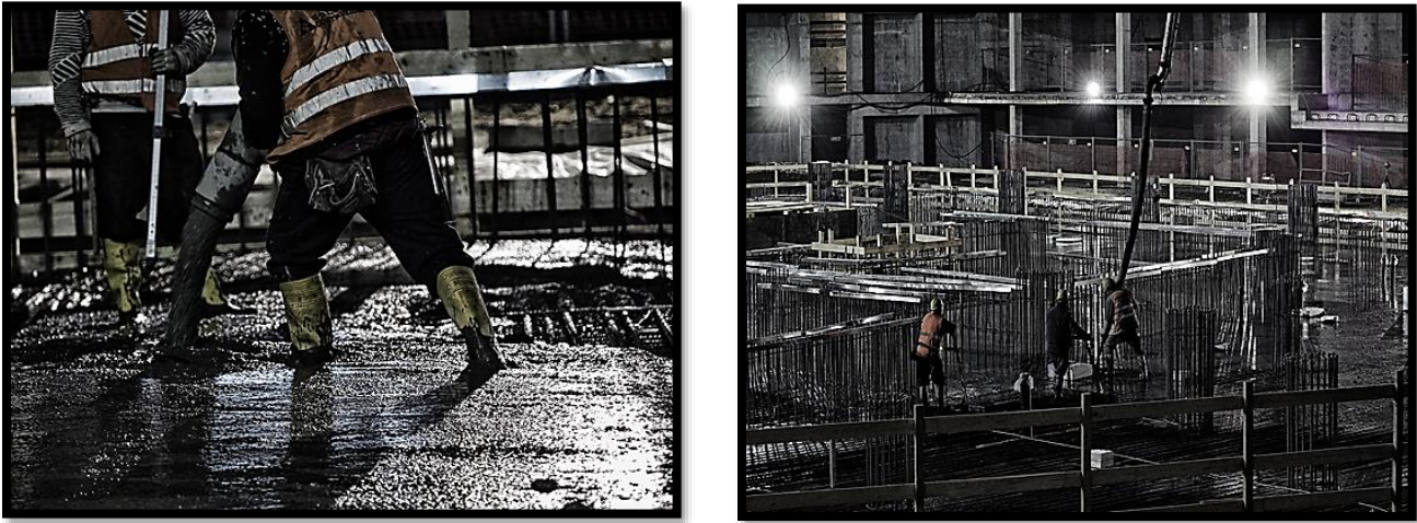
Figure 2. Getto Fondazione Torre Libeskind, Casting 22 . (Source: Holcim, 2015)
