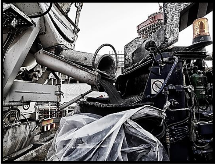
Figure 3. Getto Fondazione Torre Libeskind, Pumping concrete 22 . (Source: Holcim,2015)
