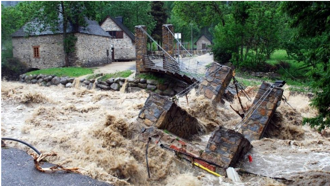
Figure 34 Destroyed bridge over the Garona river in Salardù, Vall d'Aran 7
