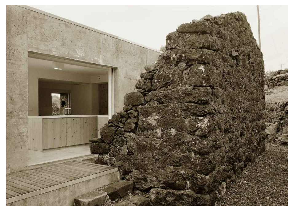
Sami-Architects, E/C House
