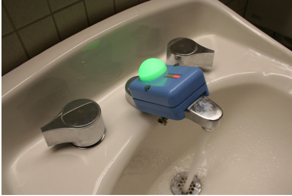
Fig. 1 Upsteam project (Kuznetsov and Paulos, 2010).
