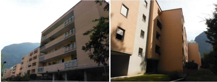
Figure 47 – Building case study_North-West façade (left) and South-East façade close to the mountain (right)
