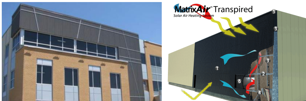
Figure 21 – Group Dion building with MatrixAir TR © façade system
