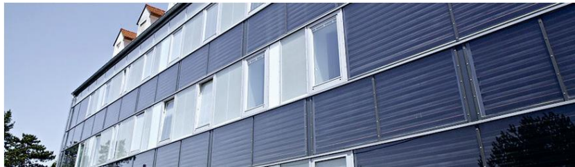
Figure 18 – GAP:water façade system installed in Austria [Source: IEA Annex 50]
