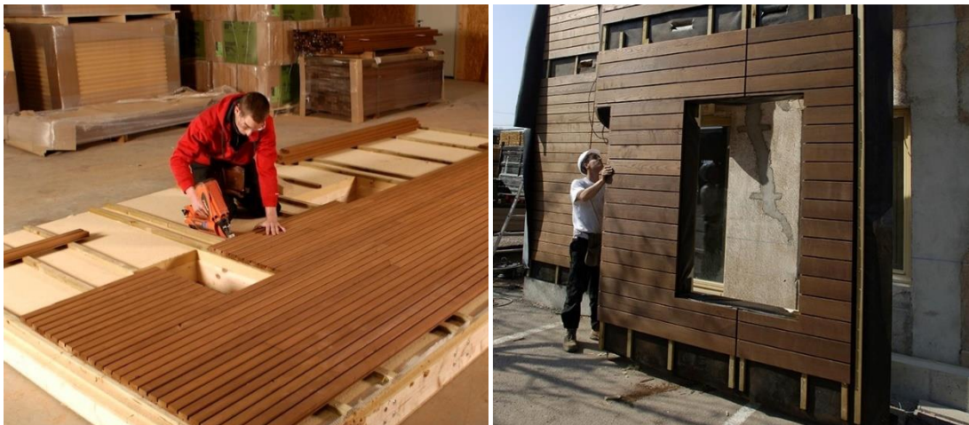
Figure 2 - Prefabricated passive façade modules (source: I-Tech-Bois [13])
