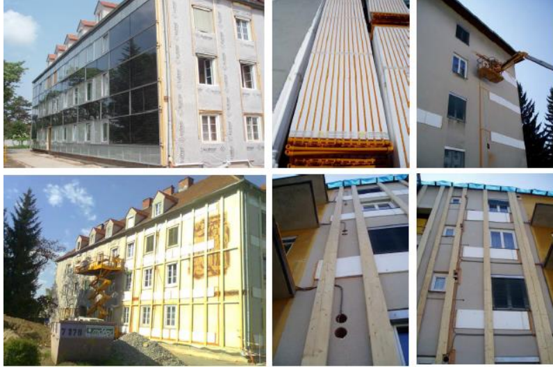
Figure 15 - Distribution system applied to the existing façade (source: AEE Intec, 2012)
