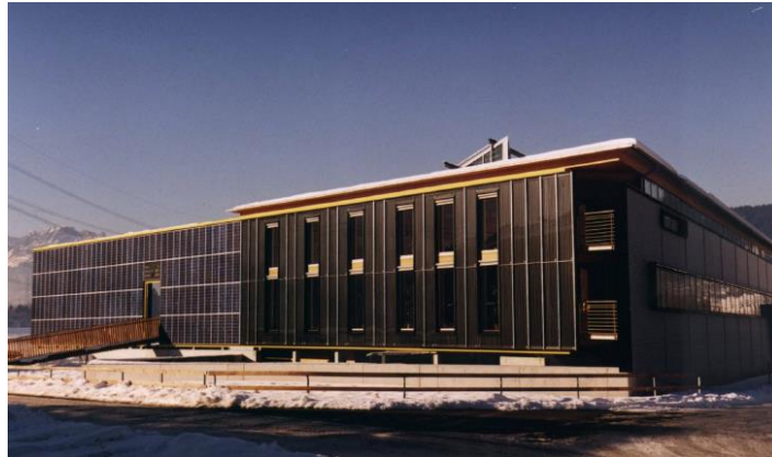
Figure 20 – AKS DOMA HQs; south oriented façade
