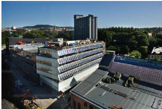
Figure 19 – Bellona Building with tilted solar envelope
