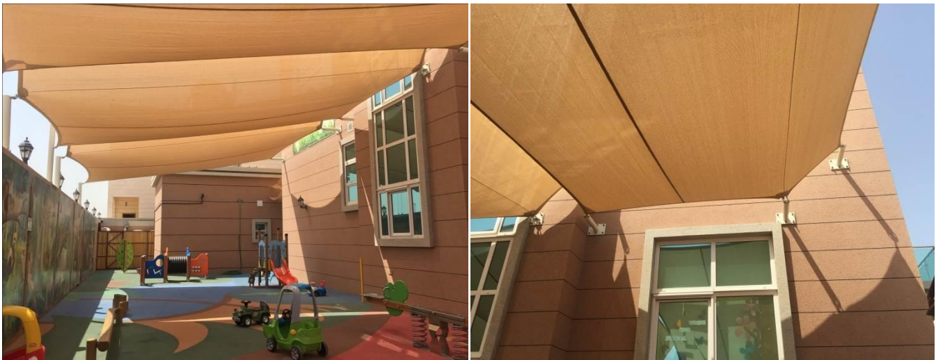
Figure 44: Site application of the shading device.
