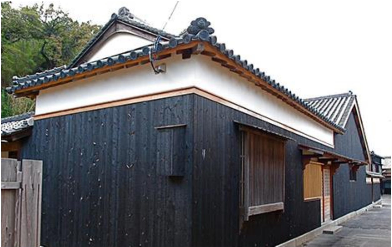
Fig. 5.3.4 House in Naoshima
