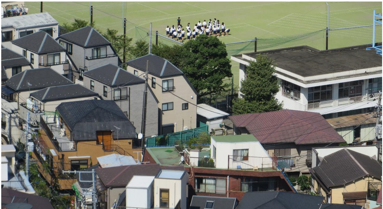
Fig. 3.1.13 Architecture disorder in a residential area
