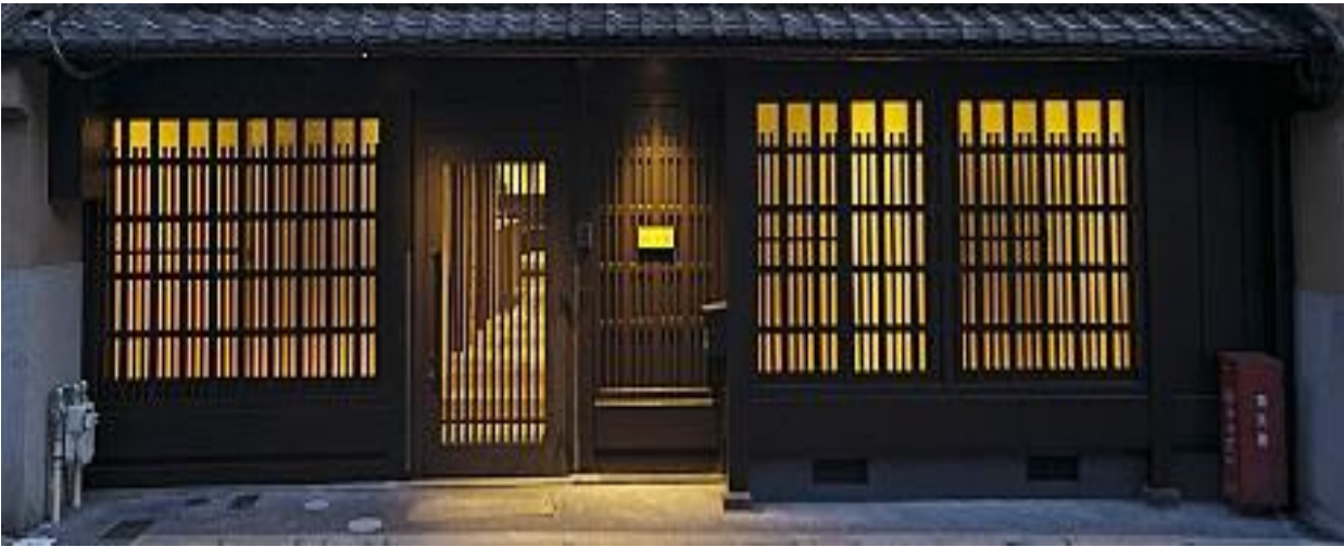
Fig. 5.3.6 Facade wooden details
