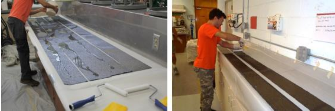
Figure 5.14 - CFRP Sheet impregnation process
