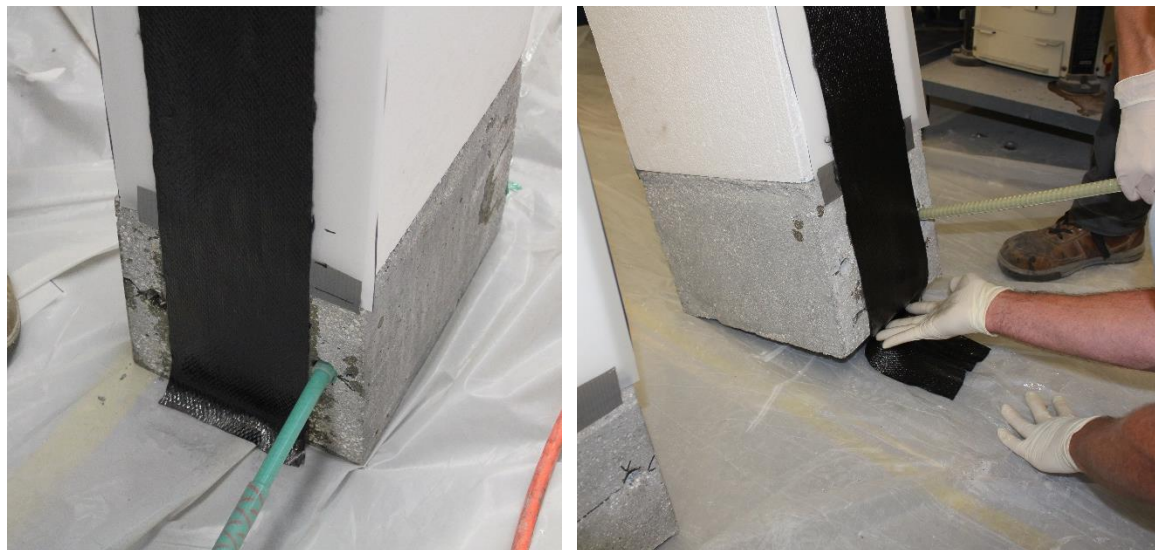
Figure 3.12 – Block's "Failure side" (left) & "Un-failure side" (right)
