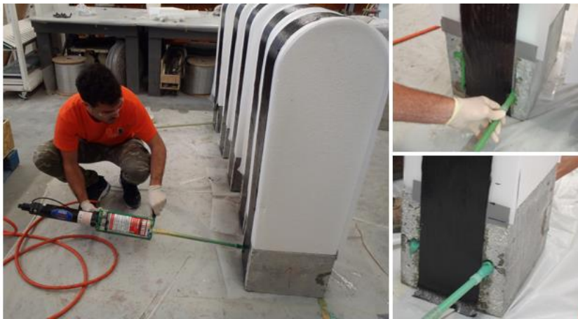
Figure 3.13 - Epoxy pouring process
