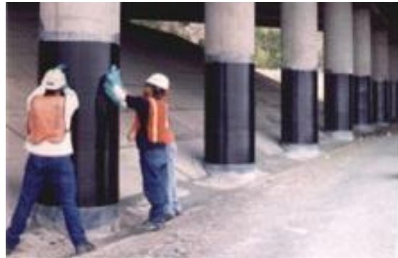
Figure 1.10 - Typical applications of externally bonded CFRP
