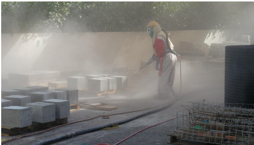
Figure 5.7 - Operation of Sandblasting
