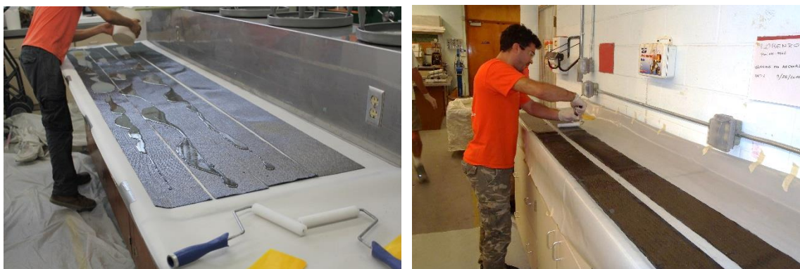
Figure 3.10 - CFRP sheet impregnation process
