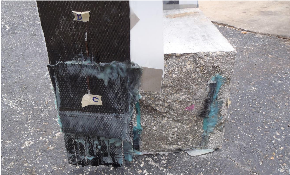
Figure 4.18 - Failure Mode D
