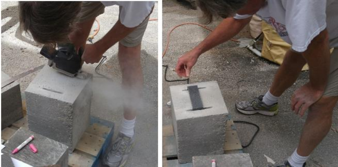
Figure 3.3 - Cutting process for the failure side of the Flat Staple anchors
