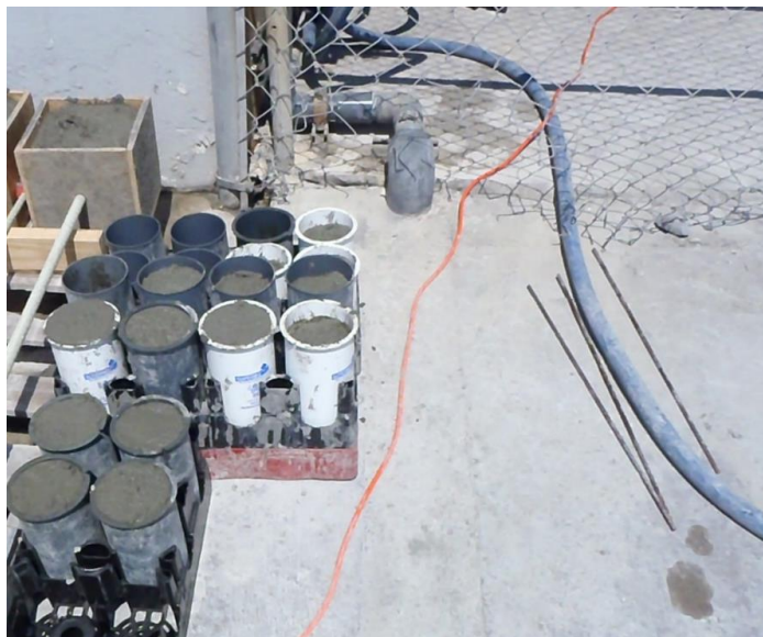
Figure 3.30 – Casting of the cylinders
