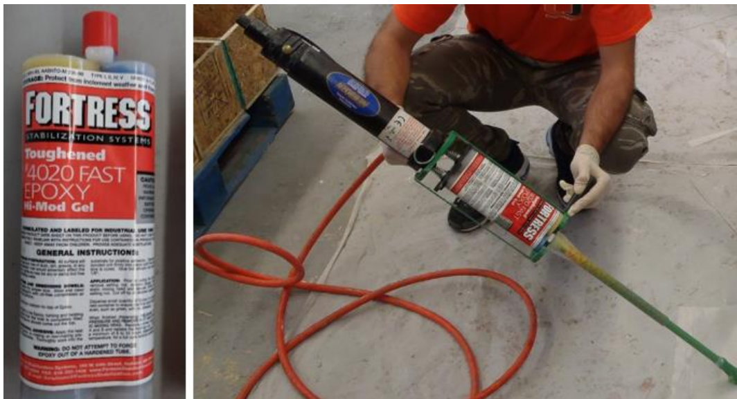
Figure 3.41 - Fortress 4020 Fast Epoxy Hi-Mod Gel & the specific epoxy gun working with compressed air
