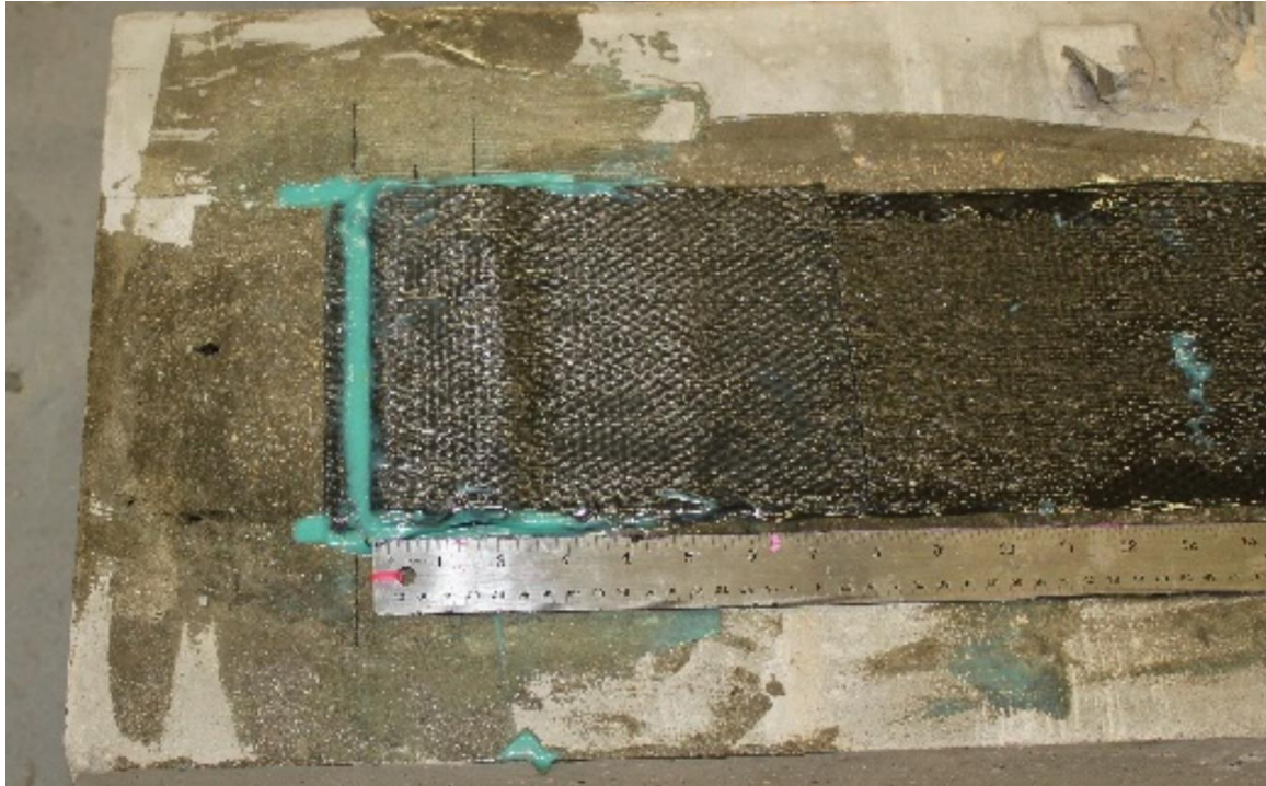
Figure 5.17 - Final product of a Flat staple anchor on slab
