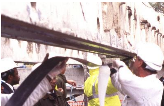
Figure 1.10 - Typical applications of externally bonded CFRP
