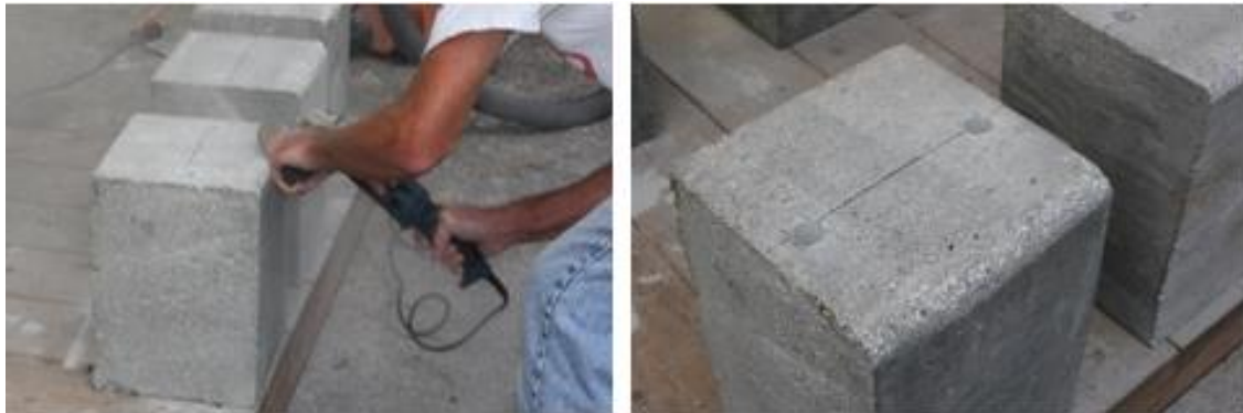
Figure 3.5 – Blocks' edge smoothing process
