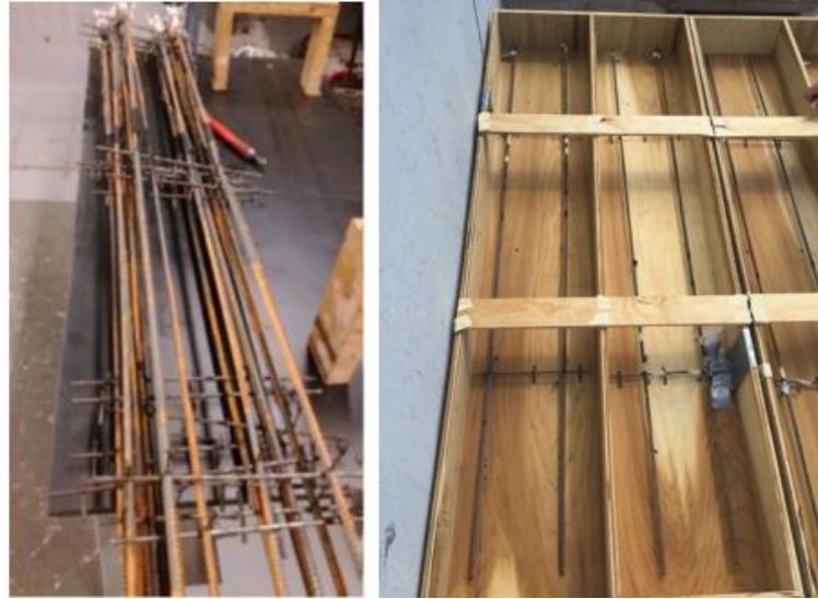
Figure 5.5 - Mold set-up
