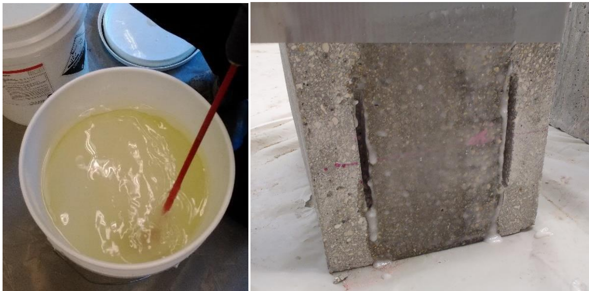
Figure 3.8 - Epoxy resin mixing & fume silica application on block surface
