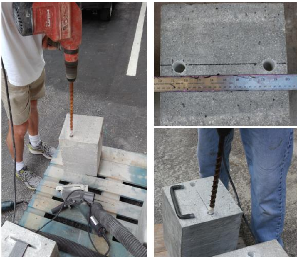
Figure 3.4 - Drilling process for the failure side of the Round Staple anchors
