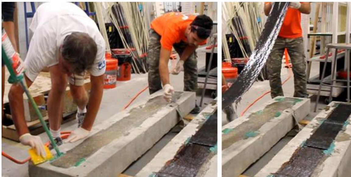
Figure 5.15 - Epoxy pouring process & impregnated FRP sheet application
