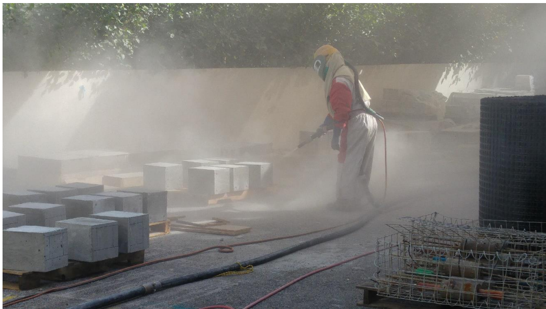
Figure 3.2 - Operation of Sandblasting
