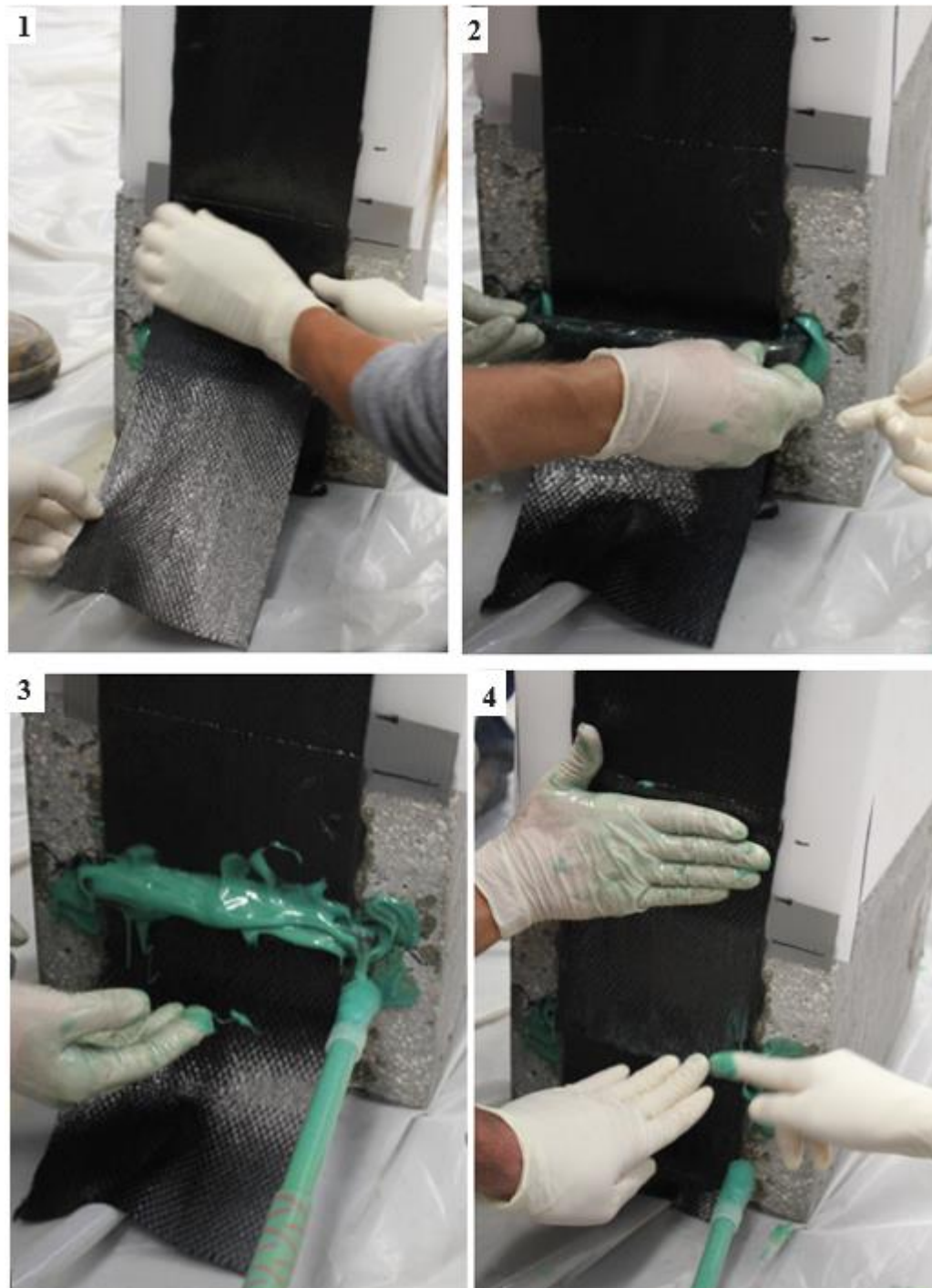
Figure 3.15 - CFRP Patch installation process
