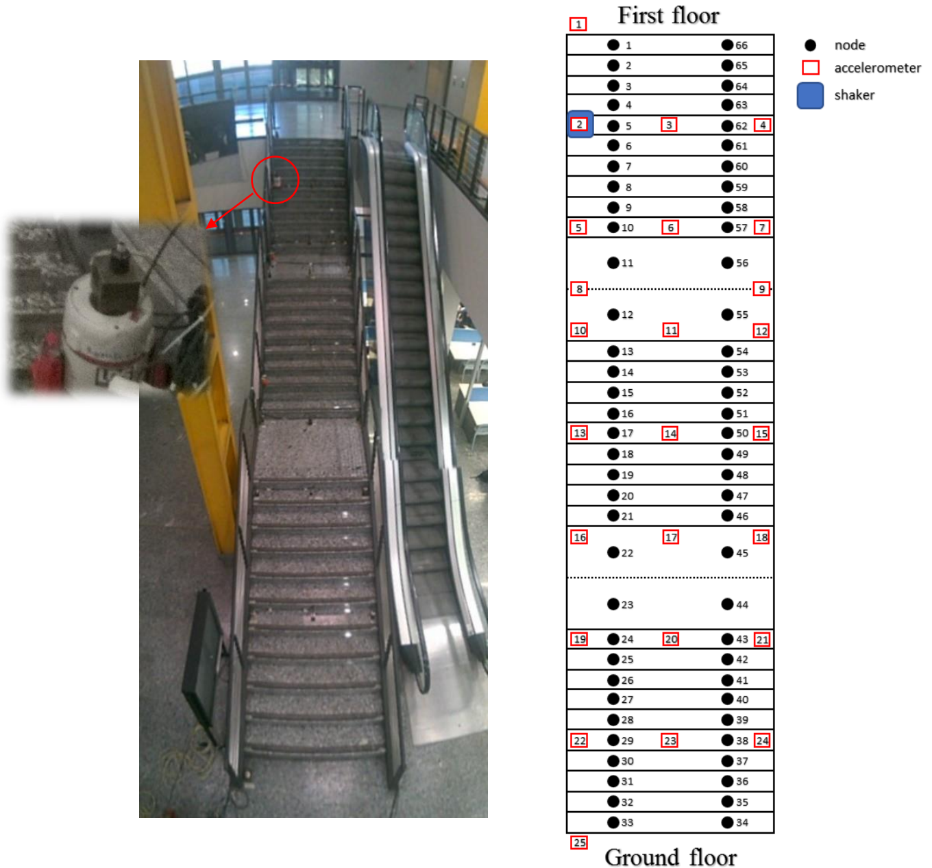
Fig. 39: Instrumented staircase (on the left) with electrodynamic shaker (small photo) and accelerometers; layout of the experimental set-up for the instrumented staircase (on the right).
