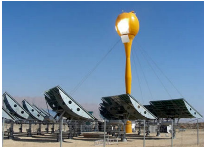
Figure 1.12 Aora plant in Spain
