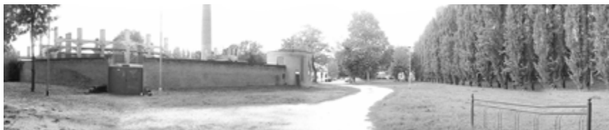
Parco U. Tognazzi, Arena Giardino e Fornace Frazzi
