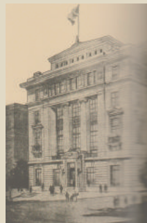
China Capital Bank Building 1923
