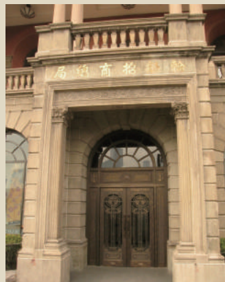
Details of the facade of the Merchants Steam Navigation Building
