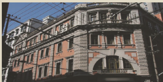
Historic Site Building
