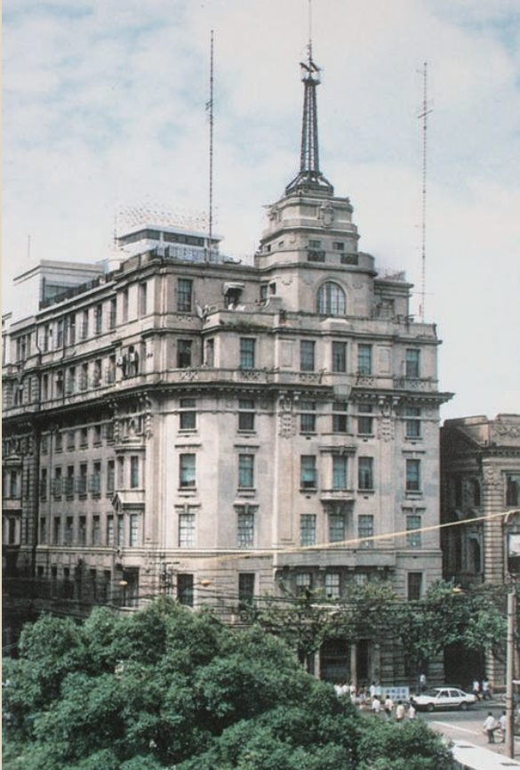
The facade of Glen Line Steamship Co. Building
