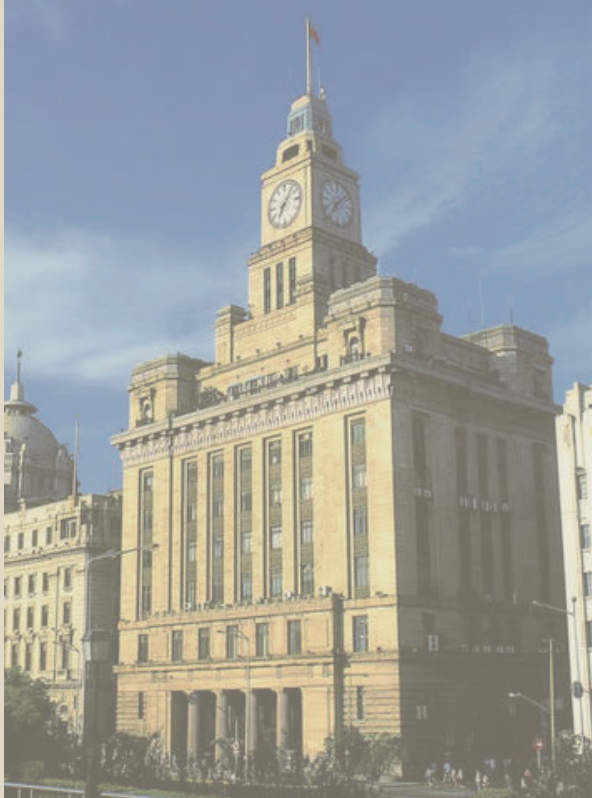
The facade of the Customs Building
