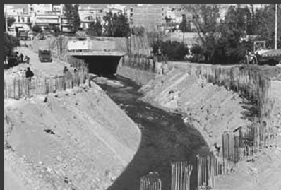
KIFFISSOS HIGHWAY CONSTRUCTION DURING '90s
