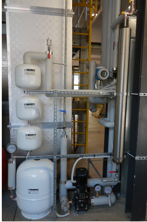
Figure 5.10: Vessel tank protection
