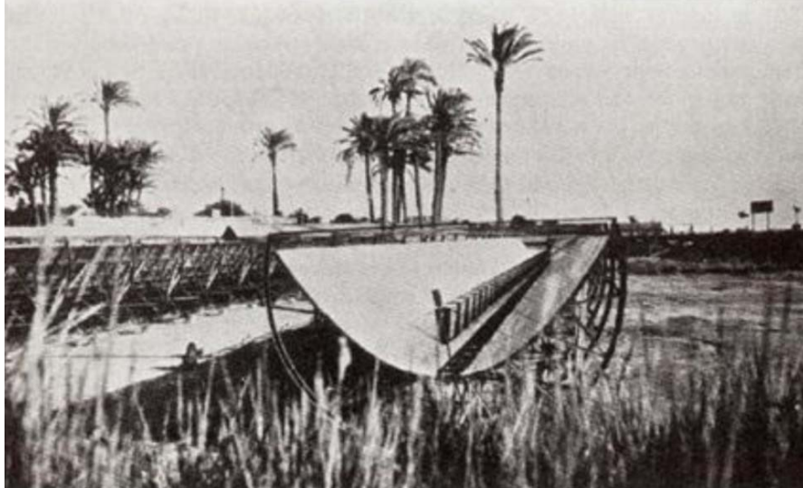
Figure 2.1: Schuman's Parabolic trough collector
