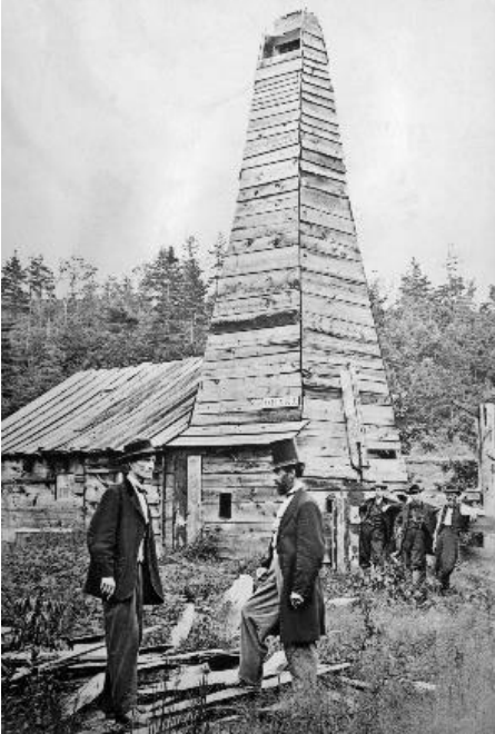
Figure A - The first oil well drilled by E.L.Drake in 1859
