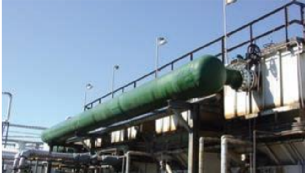
Figure 5 - Piping composite installation - courtesy of no-fiber glass system
