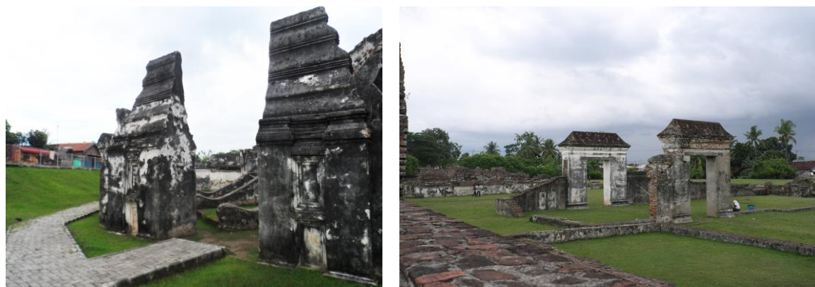
Figure 51. Ruins of Kaibon palace are in good state. (Left) Bentar /entrance of Kaibon Palace. (Right) Paduraksa entrance of Kaibon Palace.
