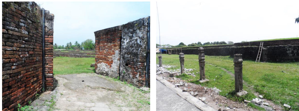
Figure 59. Two kinds of entrances: (Left) Proper and legal entrance, (Right) spontaneous and illegal entrance made by the locals using stair.
