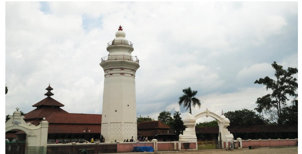
Figure 61. View of the Mosque.
