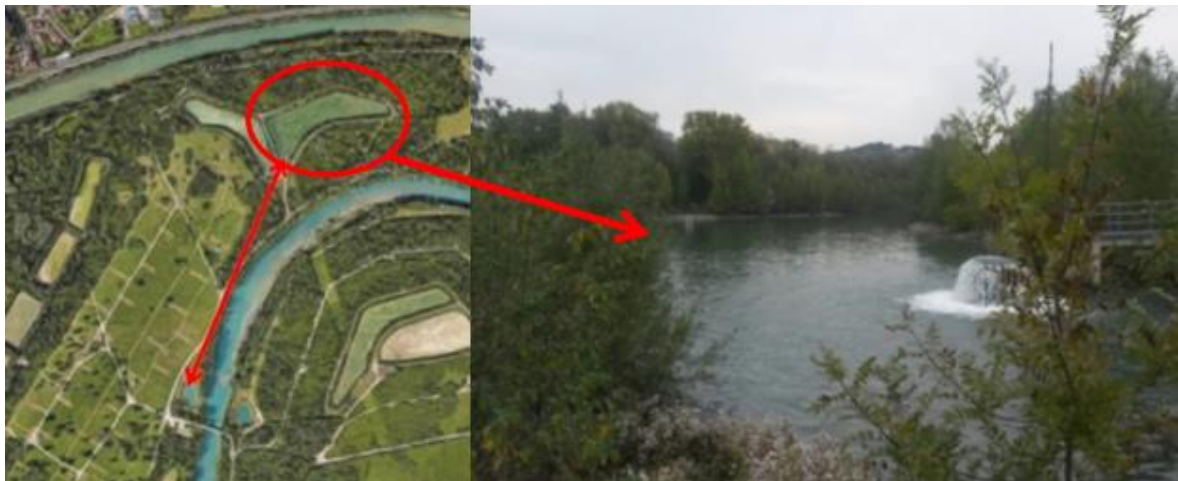
Figure 10. Pipeline to bring pre-basin's water in the infiltration basin
