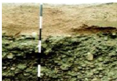
Figure 11. Section of the infiltration basins. The "filter" layer is clearly identifiable above the alluvial layers on the infiltration basins
