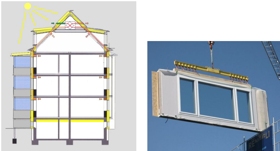
Figure 3.4: IEA EBC Annex 50. Prefabricated facade modules used to construct a new building envelope outside the existing building. (Miloni et al., 2011)
