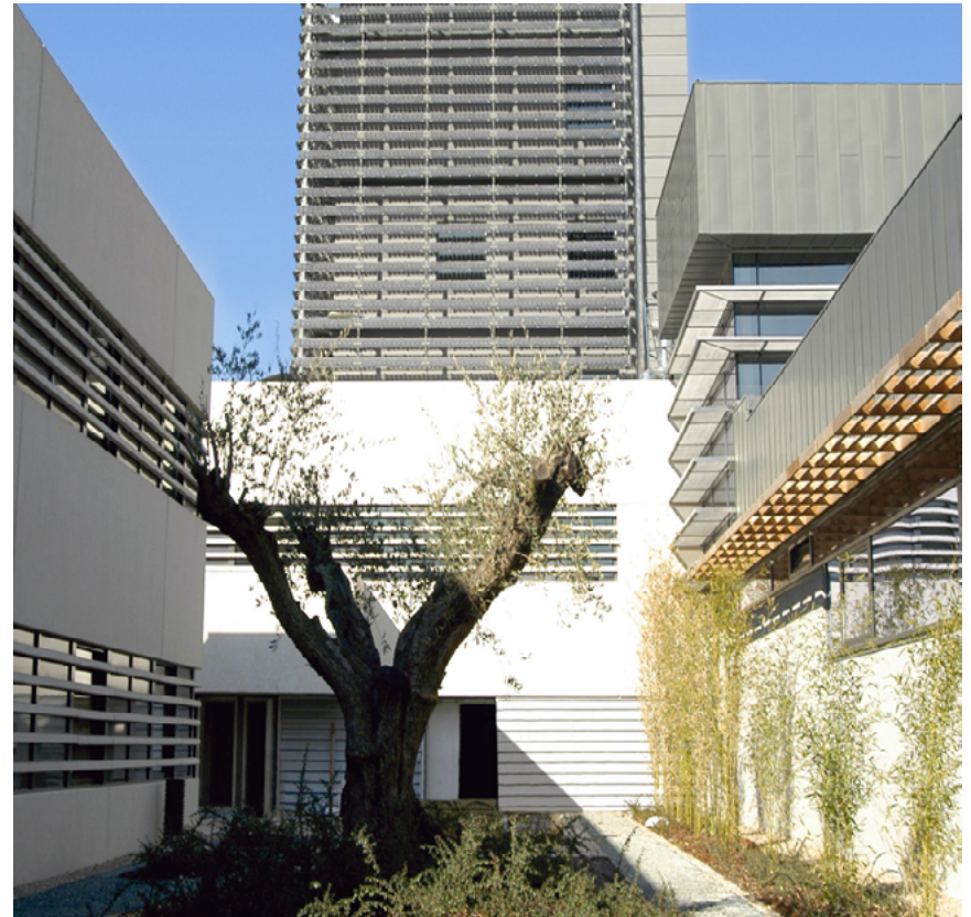
Reina Sofia foundation Alzheimer centre Estudio Lamela Arquitectos Madrid, 2006 view on the courtyard
