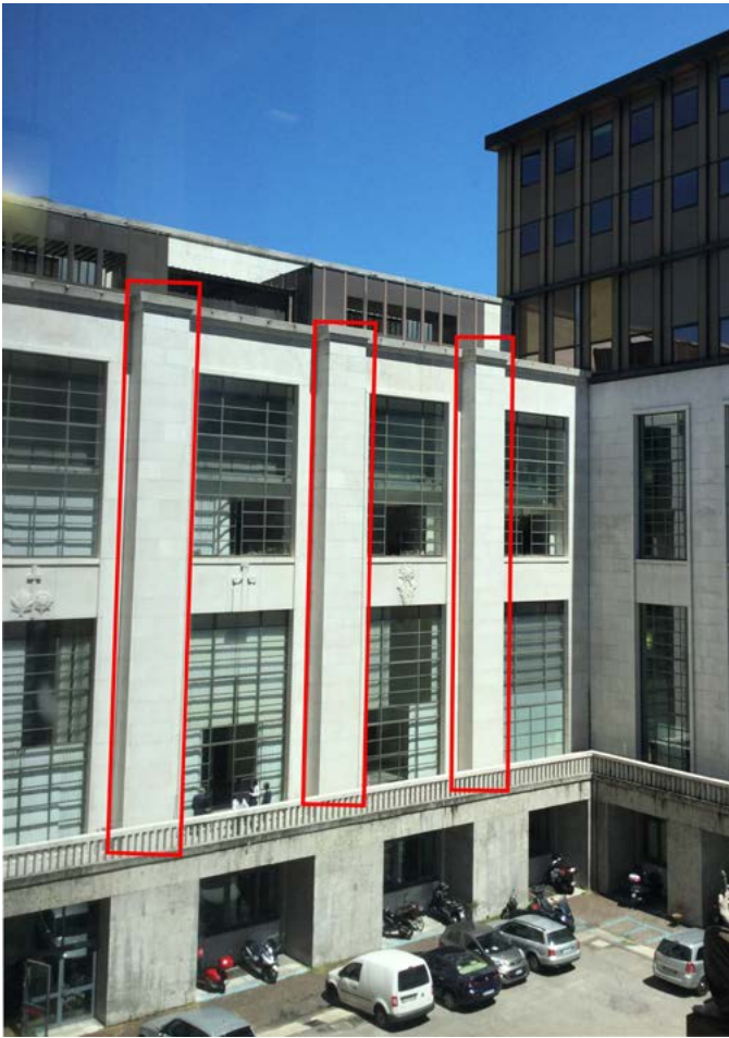
Figure 4.5.23 - Existing columns on the north facade.
