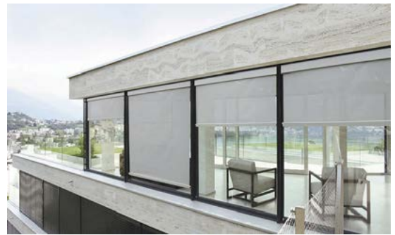
Figure 4.1.13 - Example of new installation.
