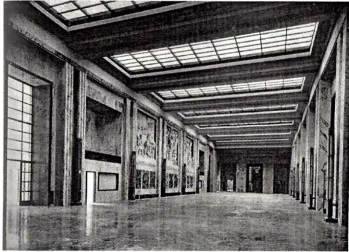
Figure 1.1.15 - Interior view of the Courthouse.
