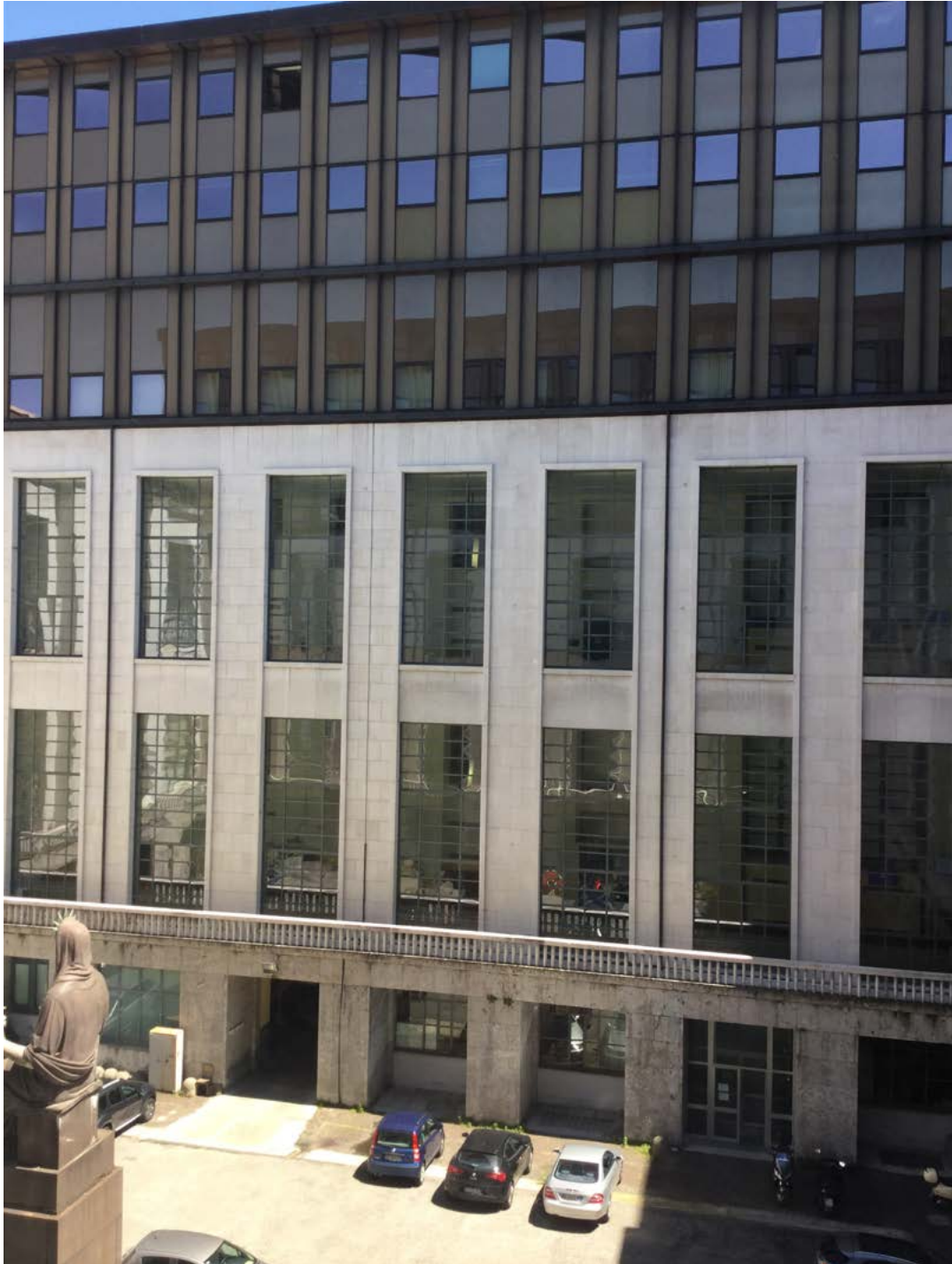
Figure 4.4.1 - View to the existing facade.
