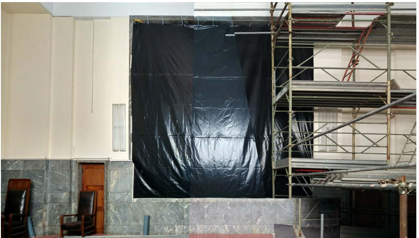
Figure 3.2.11 - Photograph of the north wall.
