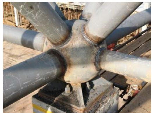
Figure 4.5.17 - Bolted vs welded sphere.
