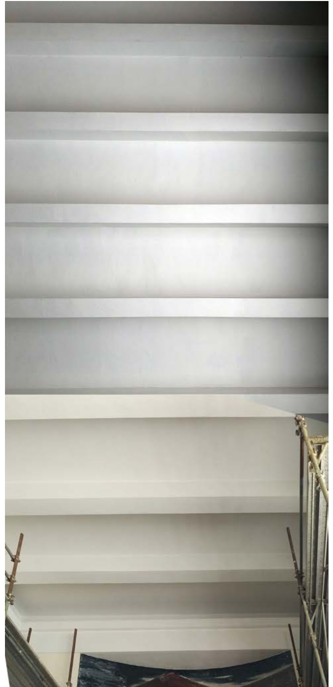
Figure 3.2.14 - Photograph of the ceiling.
