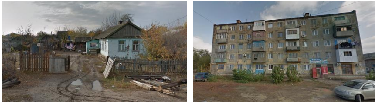
Image 4.4.10. The residential buildings in “old” Kotel’nikovo.
