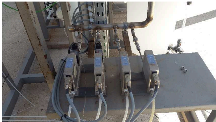
Figure 2. 6 - Burkett mass flow controller
