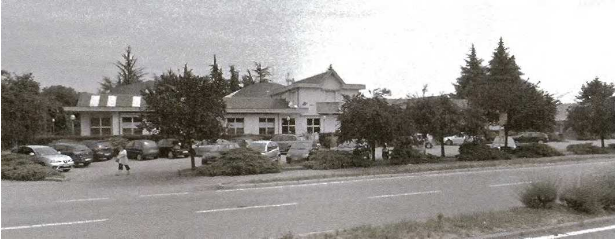
Figure 10: State of the building before the intervention
