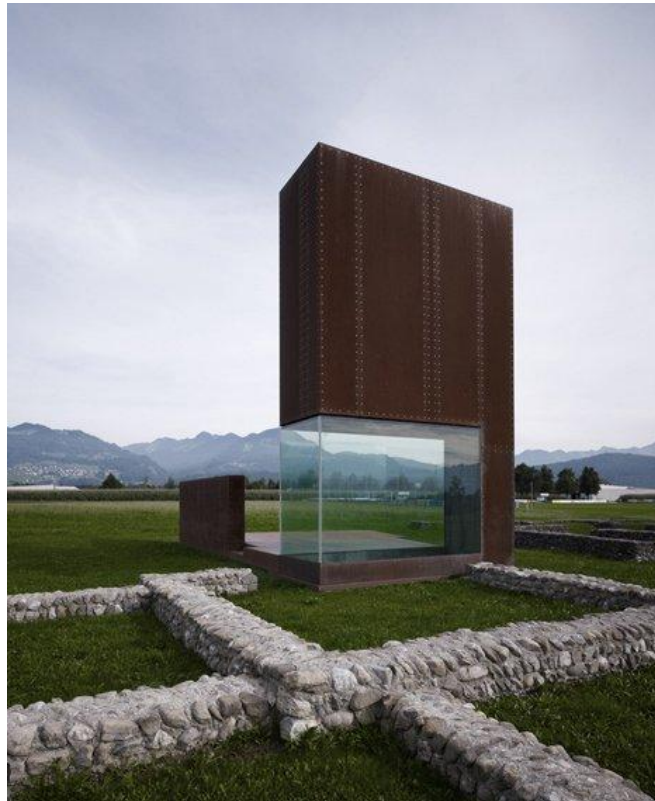
Figure 10. The use of corten steel throughout permeates the site with an historic aura and underscores the sculpted effect of the free form that helps make the excavation site a landmark.
