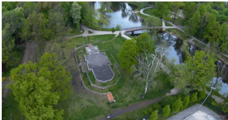
Figure 16. building site picture shot from drone
