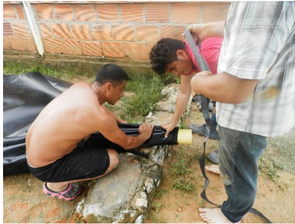
Figure 5.10 Construction of the inlet pipe.
