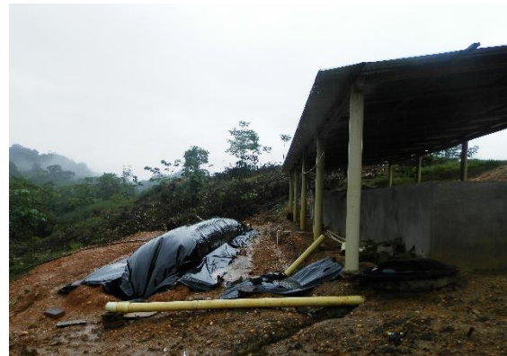
Figure 6.2 Pigsty cleaning water is now treated by the biodigester.
