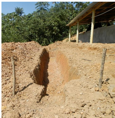
Figure 5.9 Final trench realisation.
