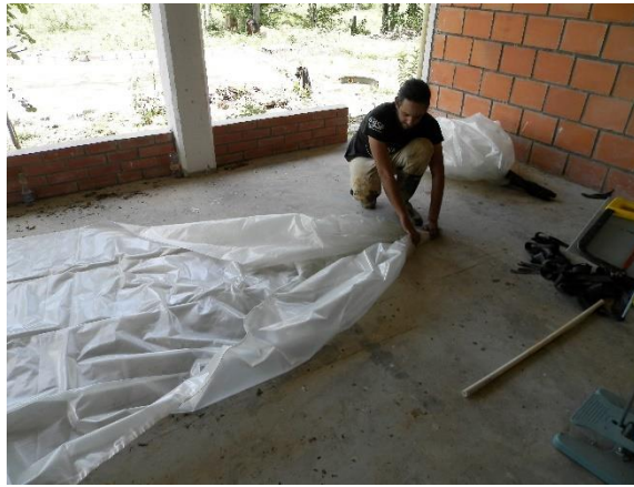
Figure 5.19 Biogas storage tanks construction phase.
