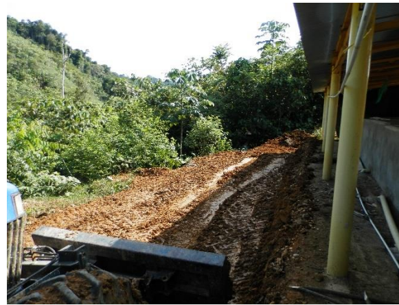
Figure 5.5 Location after the work.
