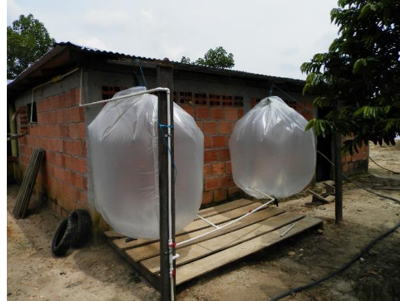
Figure 5.20 Biogas storage tanks applied on the pipeline.
