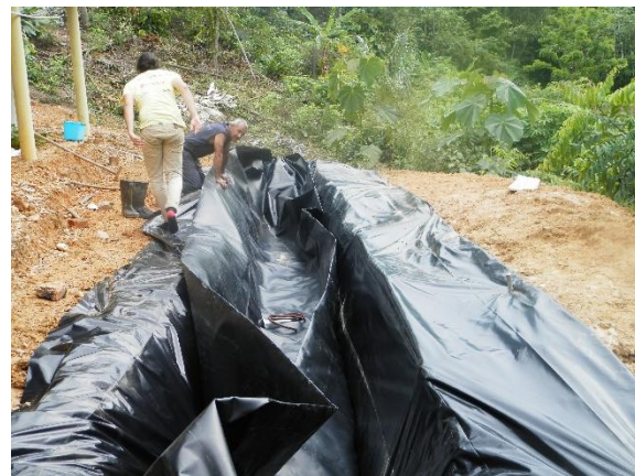
Figure 5.13 Digester bag positioning inside the trench.
