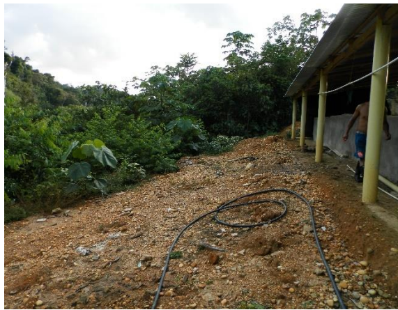
Figure 5.4 Location before the work.
