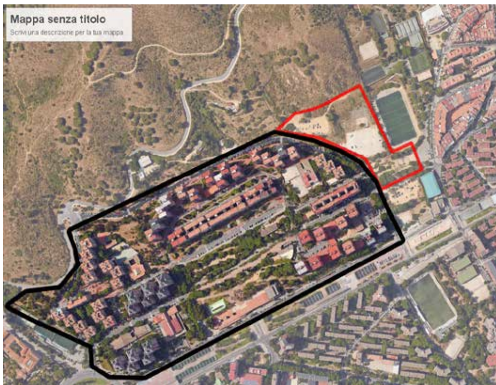
Figure 4.12 Our project site and the studied buildings in Canyelles
