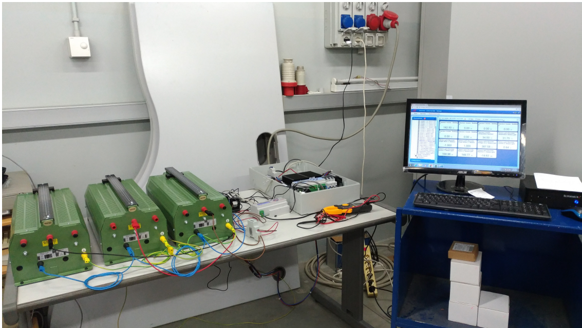
Figure D.1: Testing set-up of monitoring system: on the left, three phase load simulator, in the middle the monitoring system and on the right a PC with software Energy Sentinel Web
