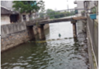
North Ren Dai Bridge
