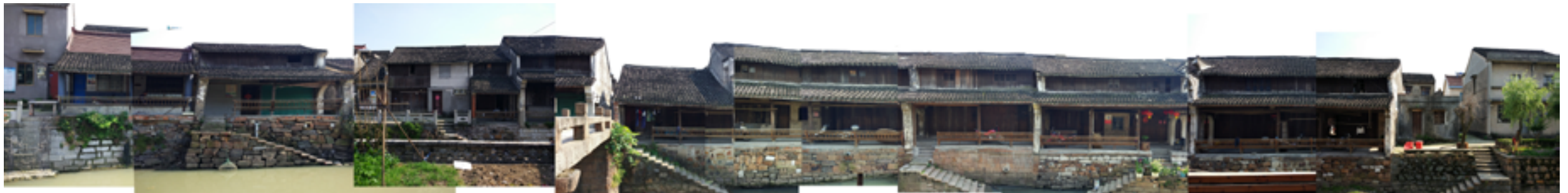
Some Part Section View of the Historical Building Photo took by Author
