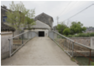
Wan Nian Bridge
