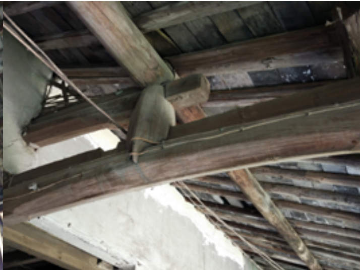
Support construction of beam Photo took by Author
