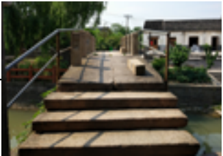
An Qin Bridge
