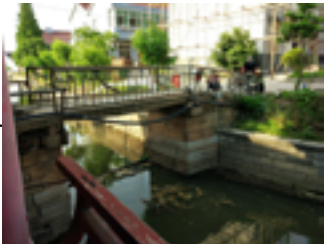
Gao Sheng Bridge
