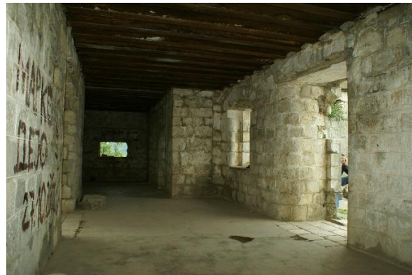
Figure 13. Artillery building; interior
