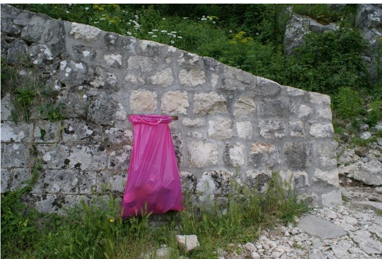
23 Example of repair intervention
