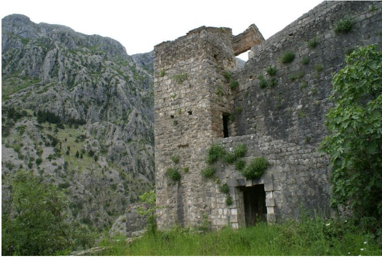
6. Contarini tower and Eastern City Gate
