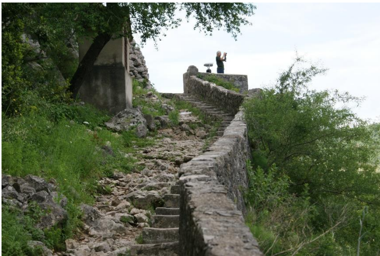
20 Main communication road and transportation ramp
