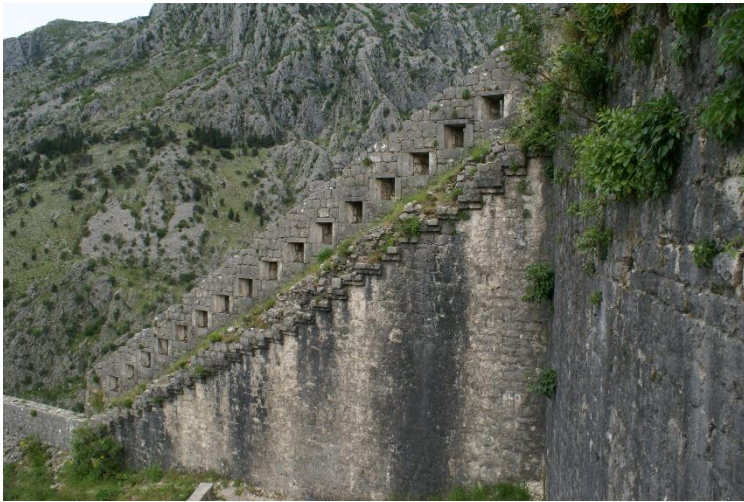
14. Medieval wall at connecting Renier and Soranzo
