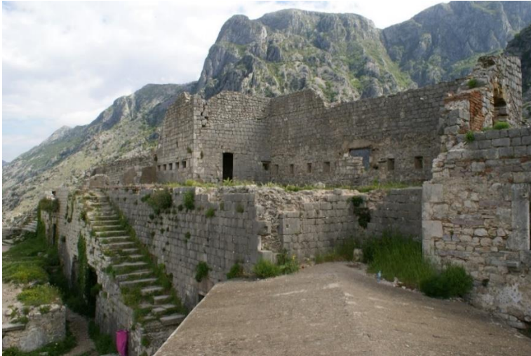
Figure 4. Platform with cistern
