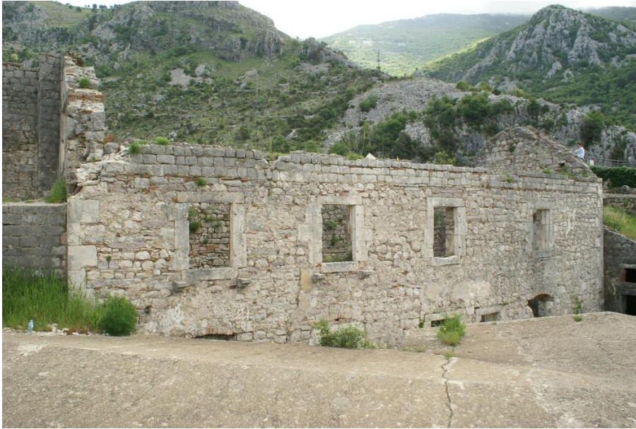
Figure 10. Main military barrack; western elevation
