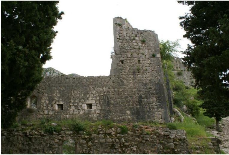
11. End of rampart path at Bataglia position
