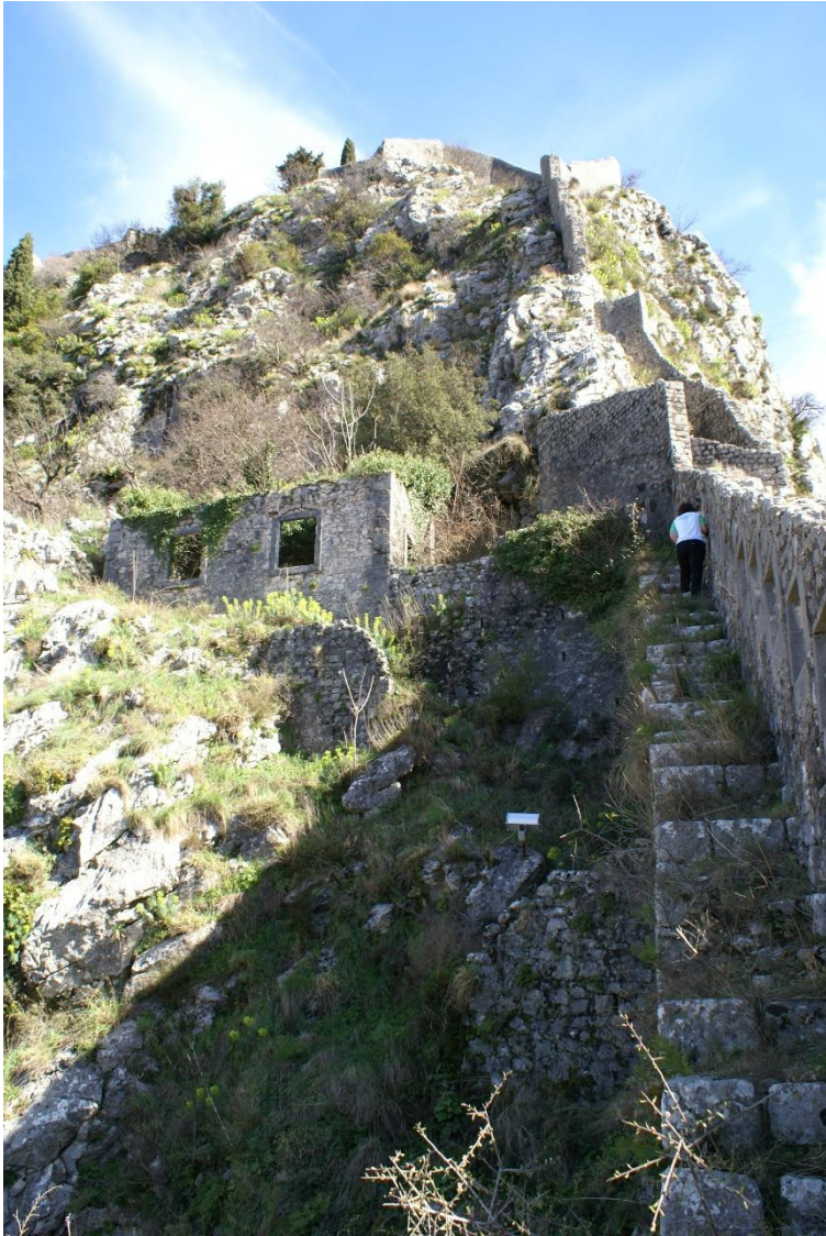
17. Rempart wall below Precipizio position
