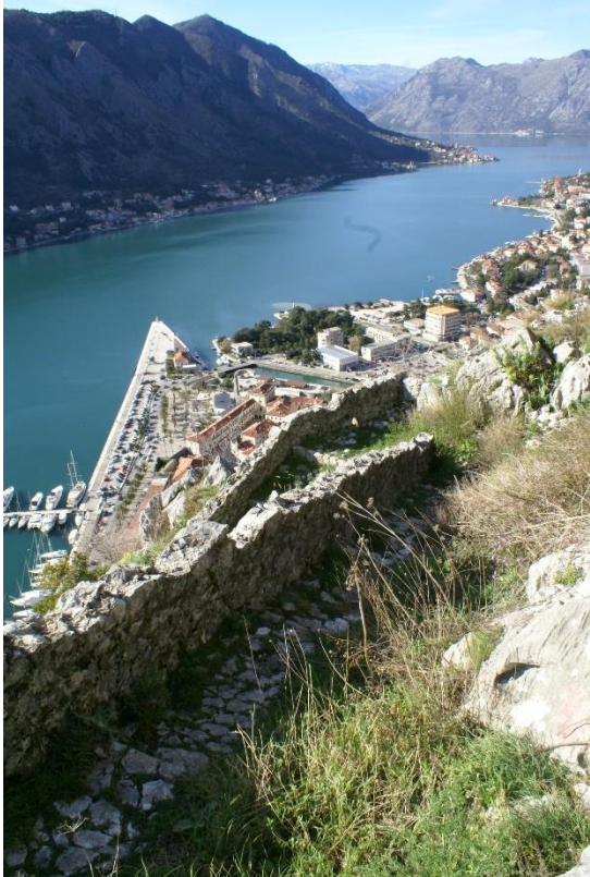
26 Maintenance and deterioration issues
