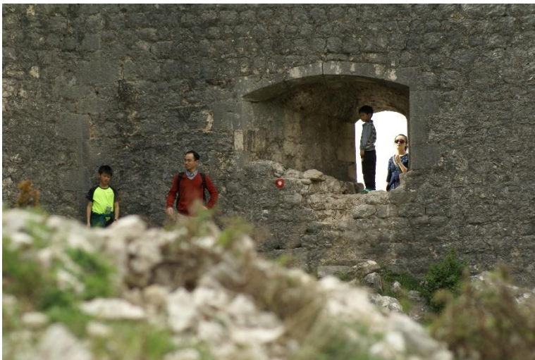
35 Artillery opening used as entrance
