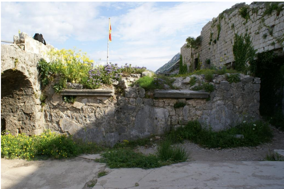
Figure 9. Remains of the "Correction house".
