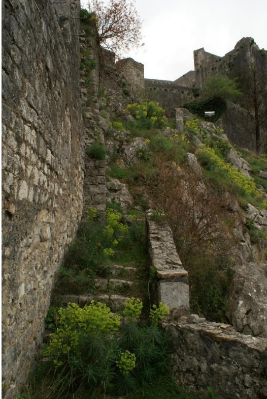
30 Neglect and bad maintenance example
