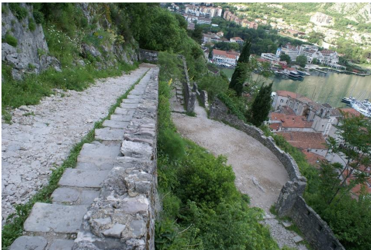
21 Main communication road and transportation ramp
